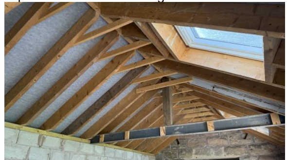
Image 4: views of the timber roof structure within B1
