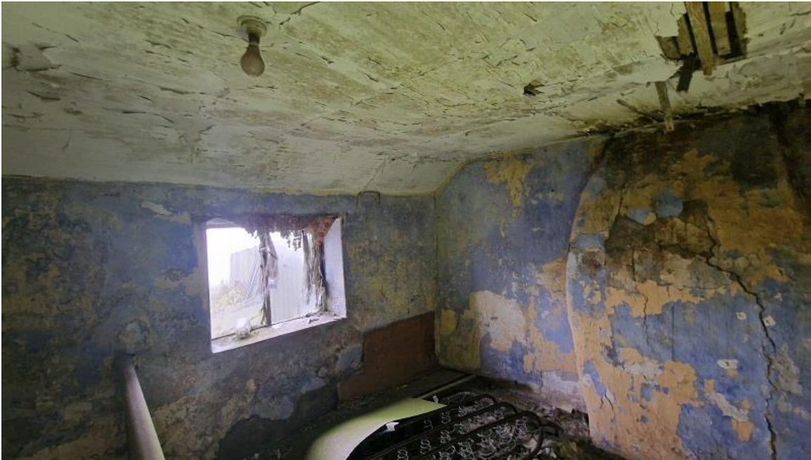
5. Upper room of farmhouse showing lath and plaster ceiling
