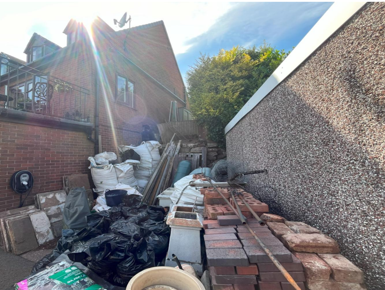
Site Photo Prince George St Cheadle.
