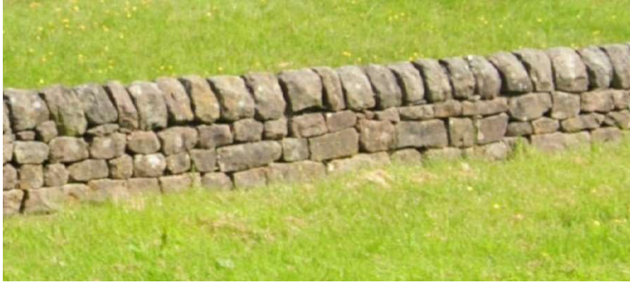
Example of dry stone wall to side of new vehicular access
