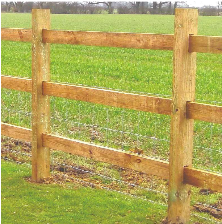
Example of post and rail fence to boundary between dwellings with hedge planted either side.
