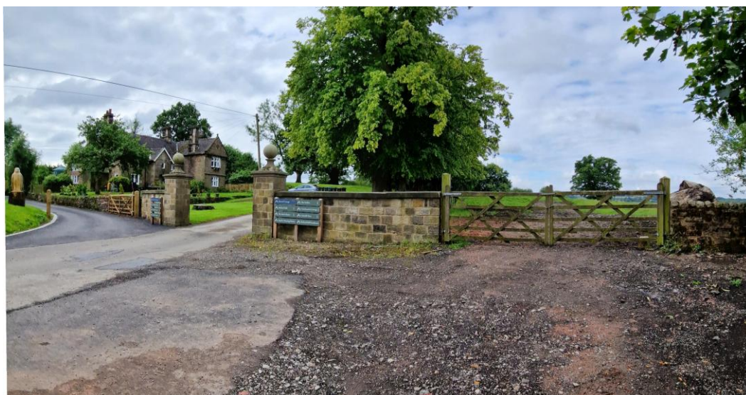
Fig.6 View of the field access gates to the proposed woodchip storage building (right), entrance to Basford Hall (left) and Lodge Cottage in the background; Source: ctd architects , 2024
