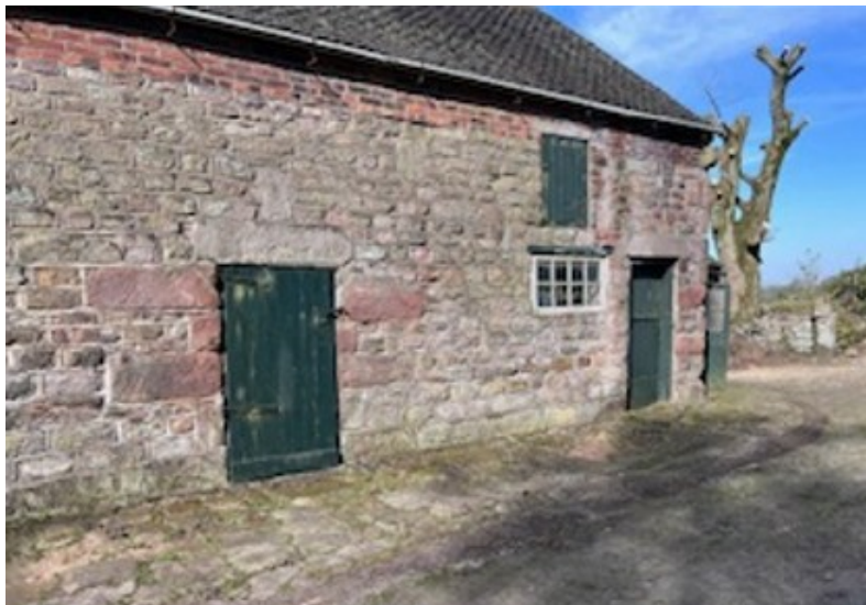
Photo 6– Barn : front elevation
