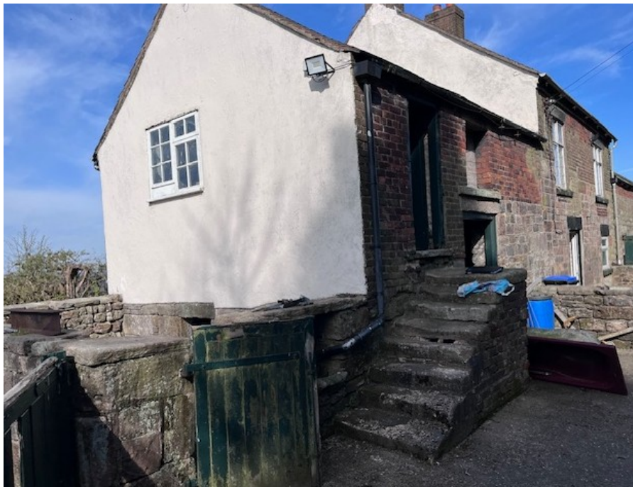
Photo 2– Coal Store : Front and Side View
