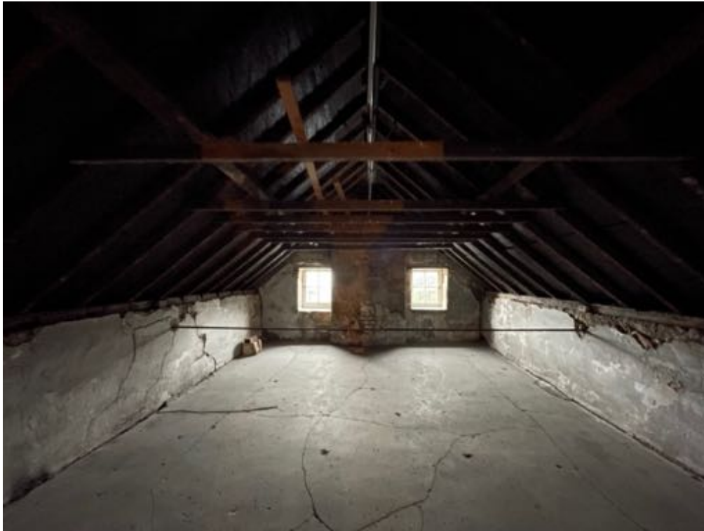
Plate 18. Room 14. Showing plaster floor, brick chimney breast and tie beam across the room.
