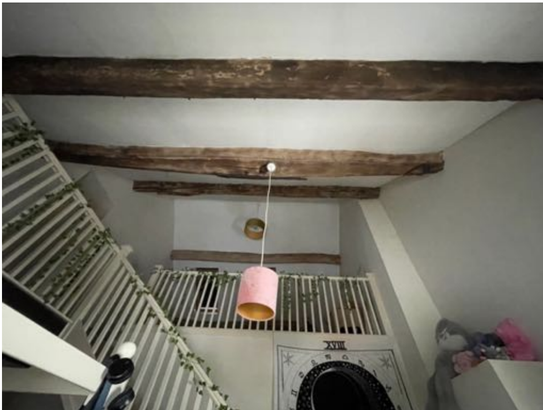
Plate 11. Room 11 in Range 3 with modern staircase to the attic space and exposed original purlins.
