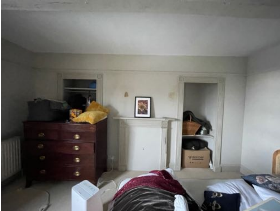
Plate 9. Room 7 in Range 1 showing moulded fire surround and decorative frames to the flanking alcoves.
