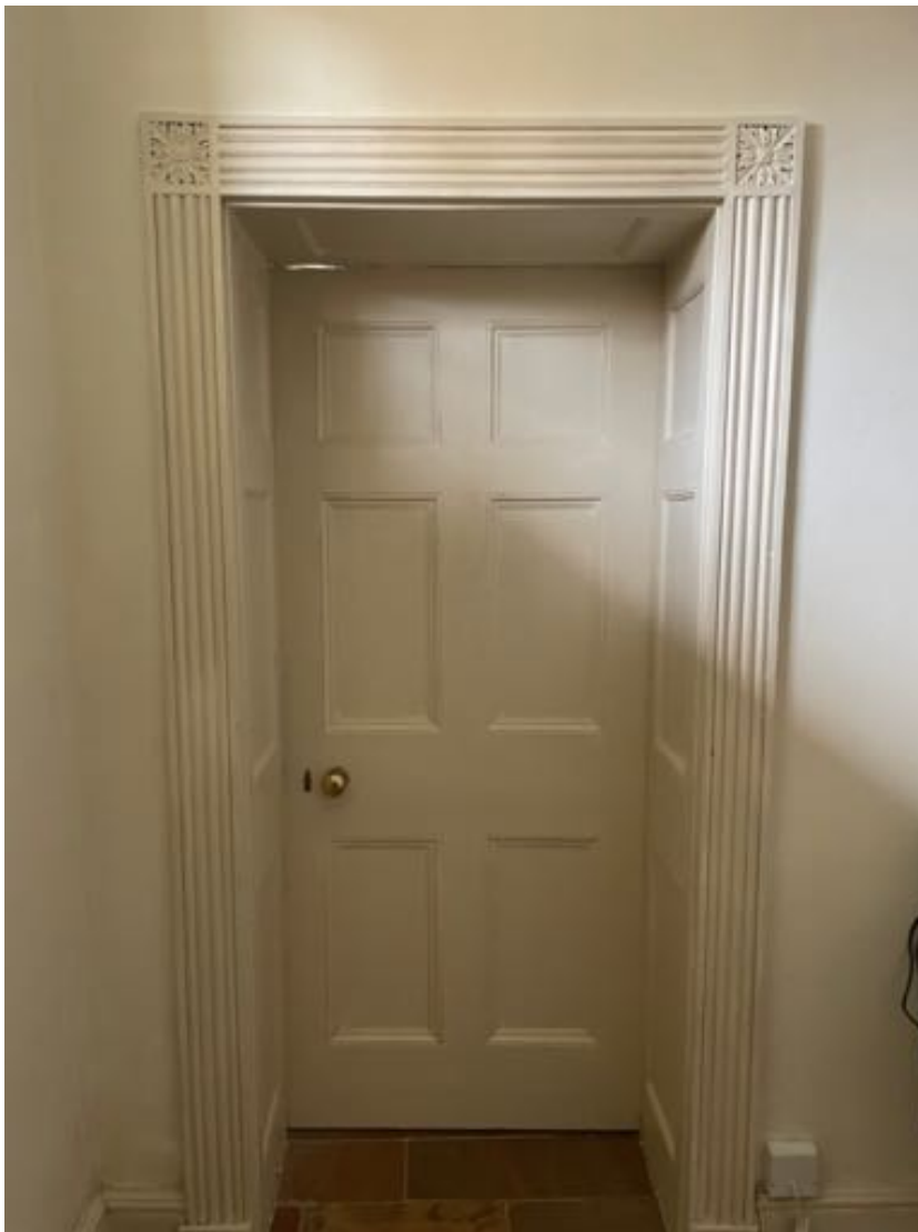
Plate 4. Example of a doorway in the entrance hall with original moulded frame, panelled recess and six-panel door.
