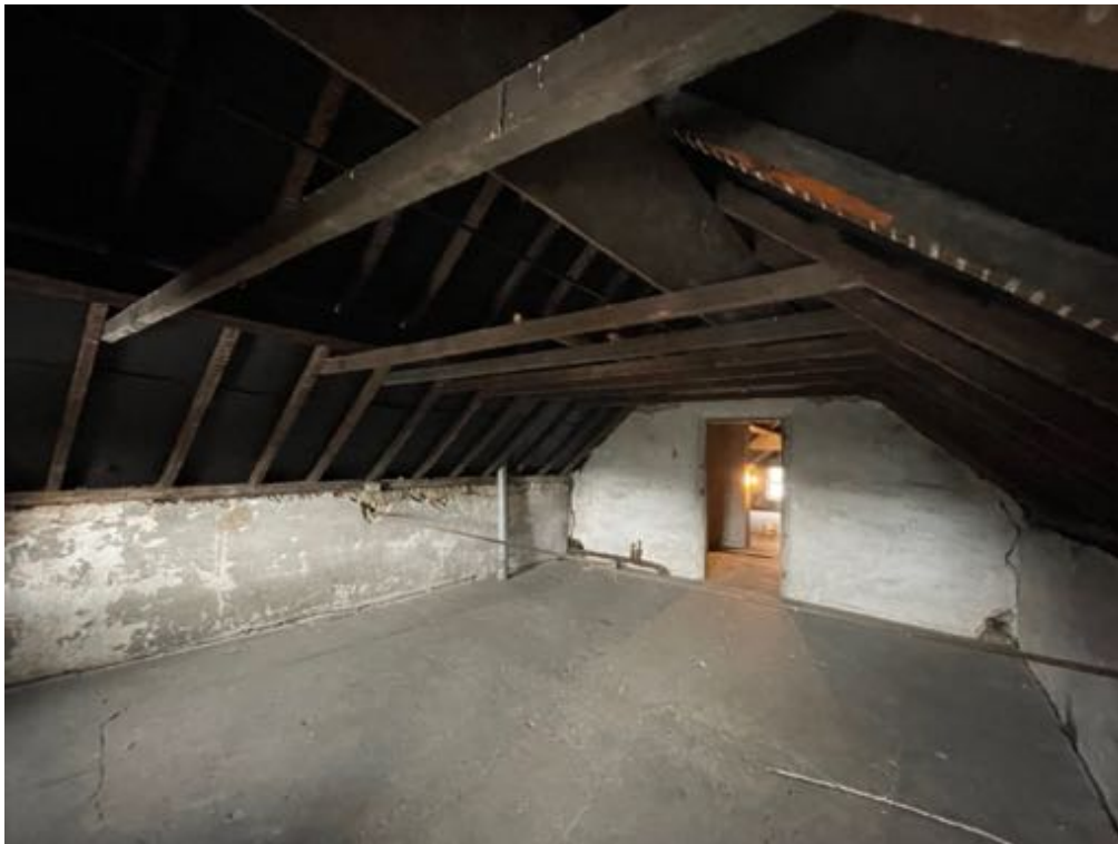
Plate 19. Room 14 showing recent/modern roof beams.
