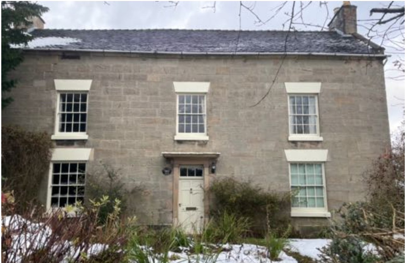
Plate 1. The front, south facing elevation of Range 1.
