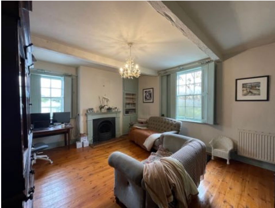
Plate 5. Room 1 showing original timber shutters and chamfered ceiling beams. The fire surround is a modern replica.
