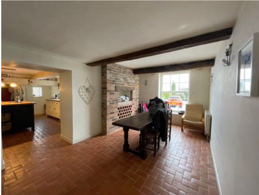
Plate 7. Room 3 in Range 2 with modified original chimney breast and chamfered ceiling beams.
