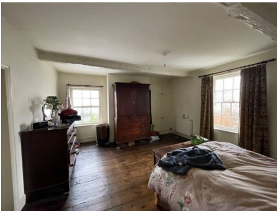
Plate 10. Room 6 in Range 1 showing chamfered ceiling beams, original floorboards and cupboard to the right of the fire breast.
