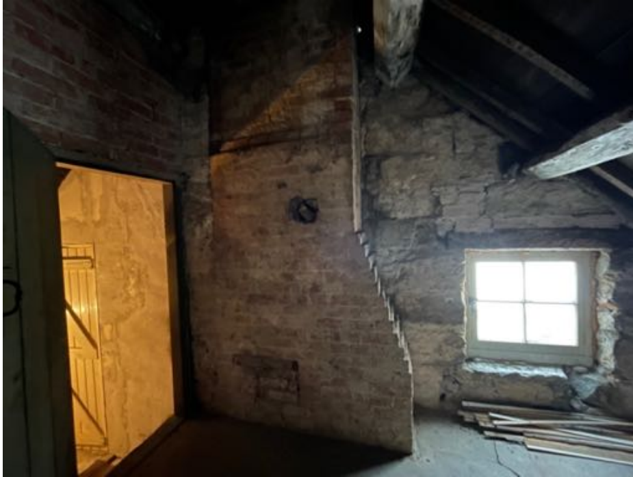
Plate 14. Brick chimney breast in Room 13.
