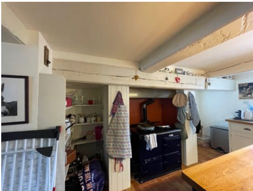
Plate 8. Room 4 in Range 3 showing inglenook with an in situ bressummer and chamfered ceiling beams.
