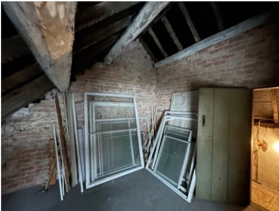
Plate 13. Room 13 in Range 2 showing brick walls and original purlins.
