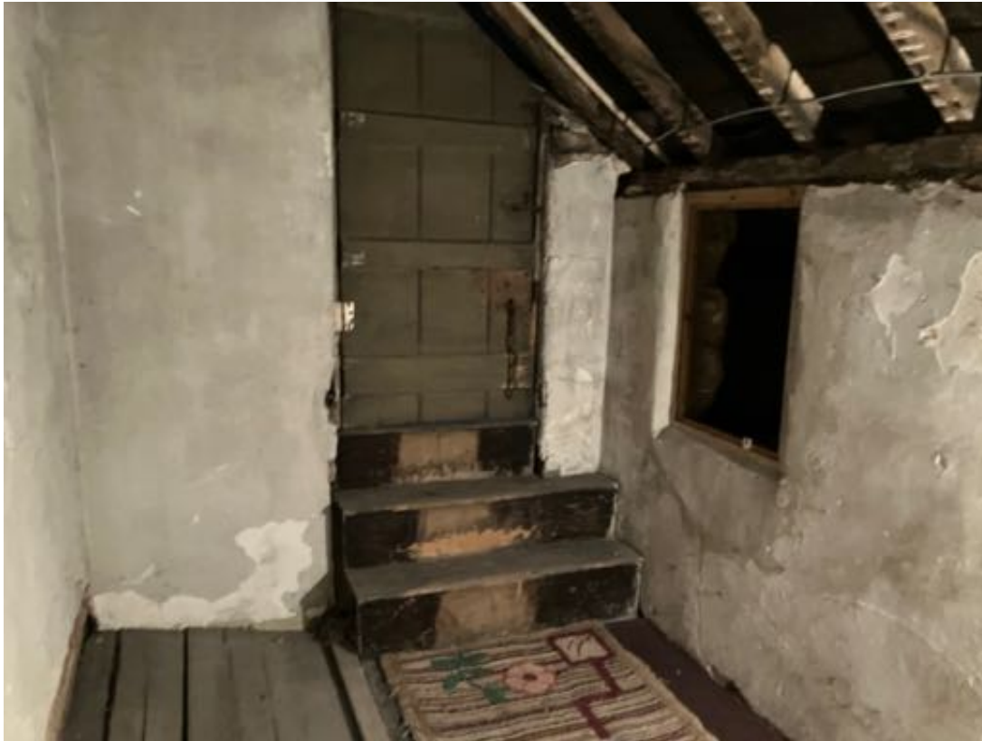
Plate 12. Room 12, showing plastered walls and loose floorboards to the left of the photograph. The door is original and leads into Room 13.
