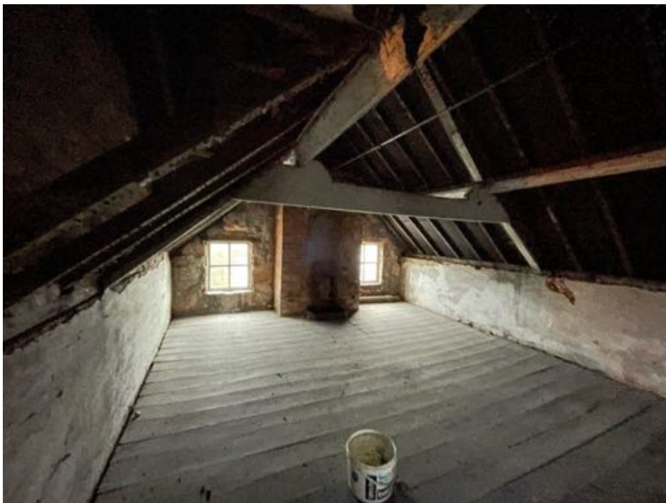
Plate 15. Room 16 showing original floorboards, brick chimney breast and recycled truss.
