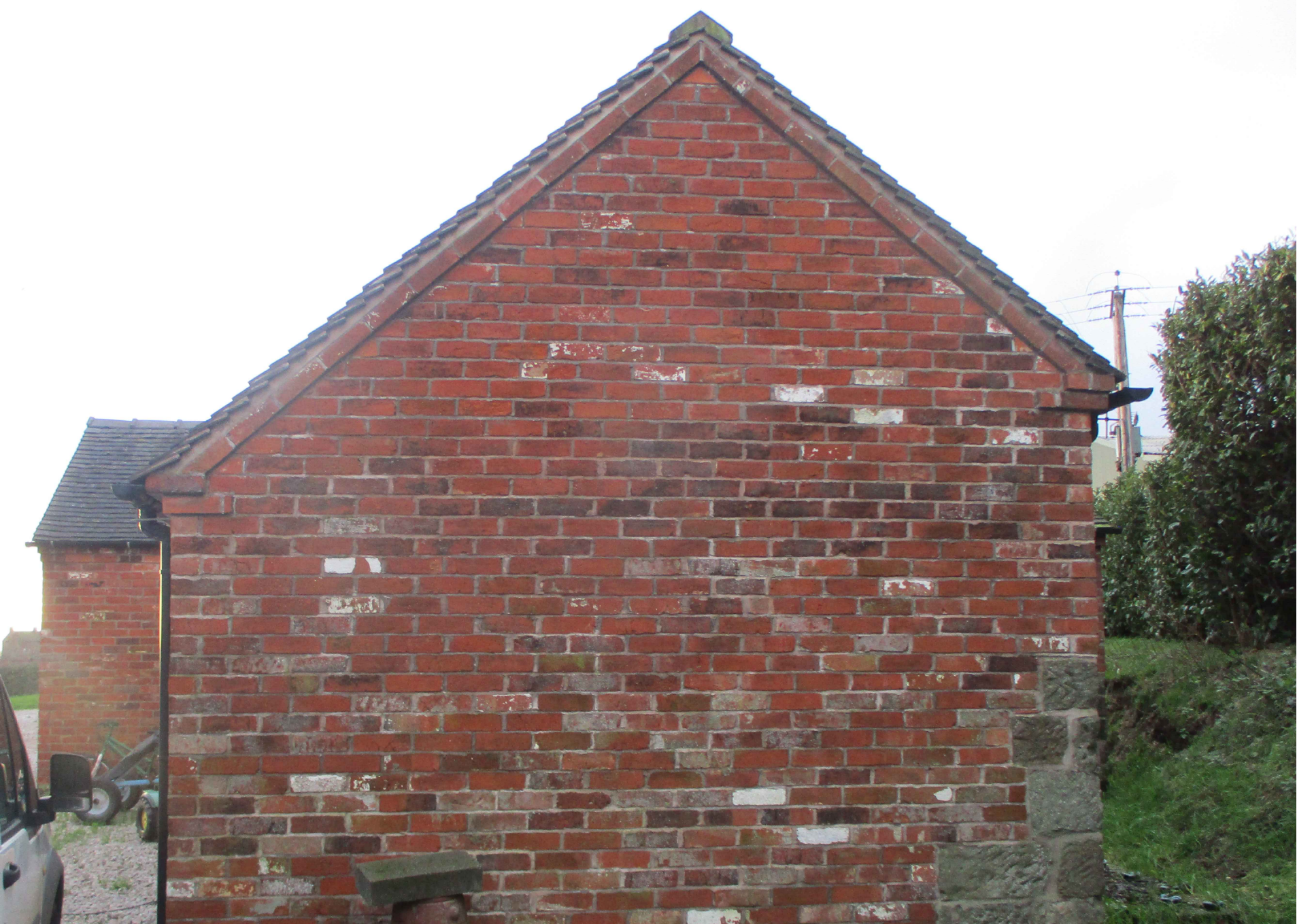
Photograph of East Elevation
