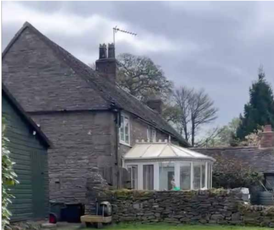
South east view of the house. There are no propose changes to this elevation.
