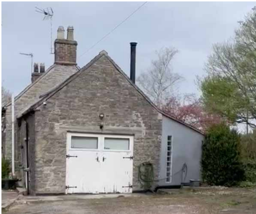
North view of the house. Location of new extension. Note that extension is to have a reduced ridge height to allow legibility of the phase of construction. Garage door to be removed.
