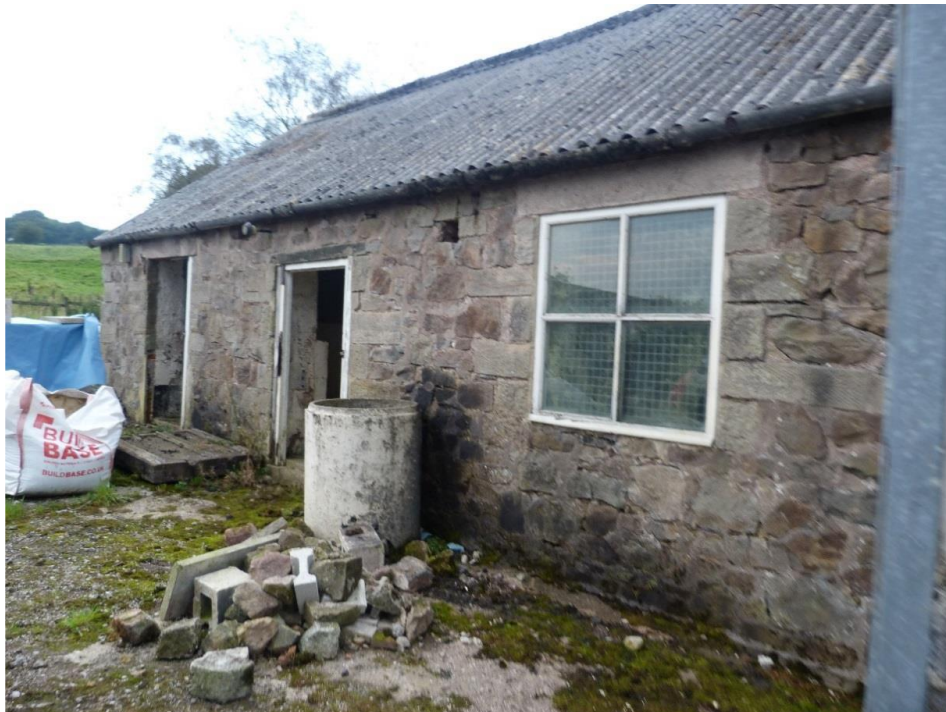
Figure 2: Stone barn prior to change of use
