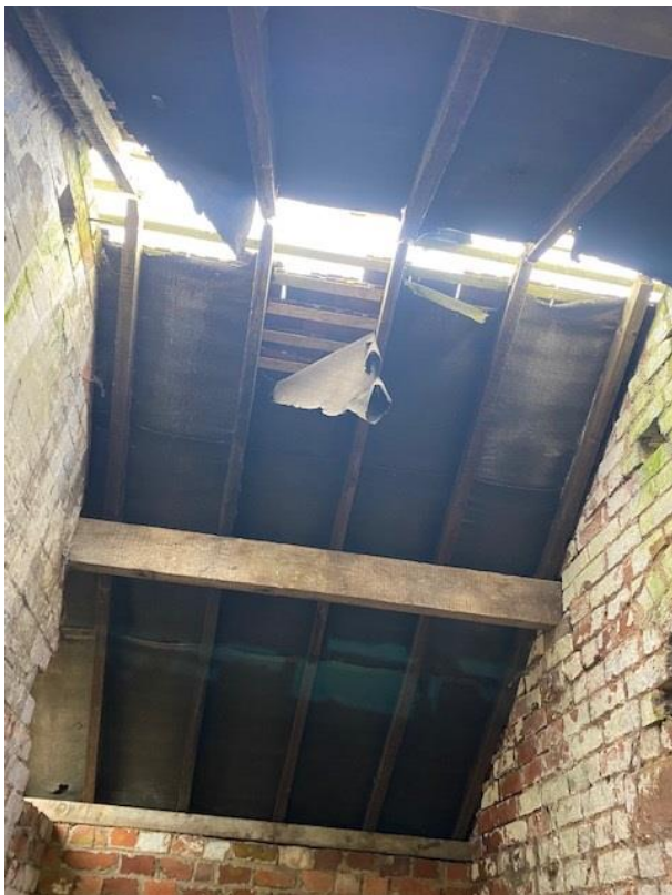
Figure 9. East elevation interior roof
