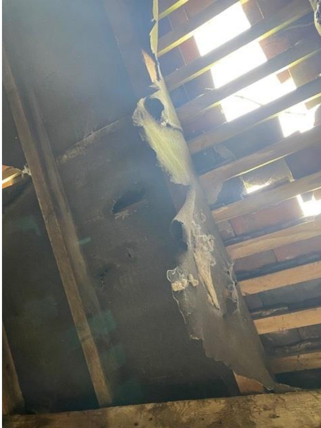
Figure 10. Western elevation interior roof condition
