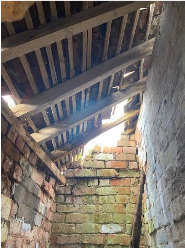
Figure 8. Interior southeast corner
