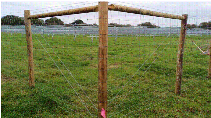
Typical example of proposed corner post array
