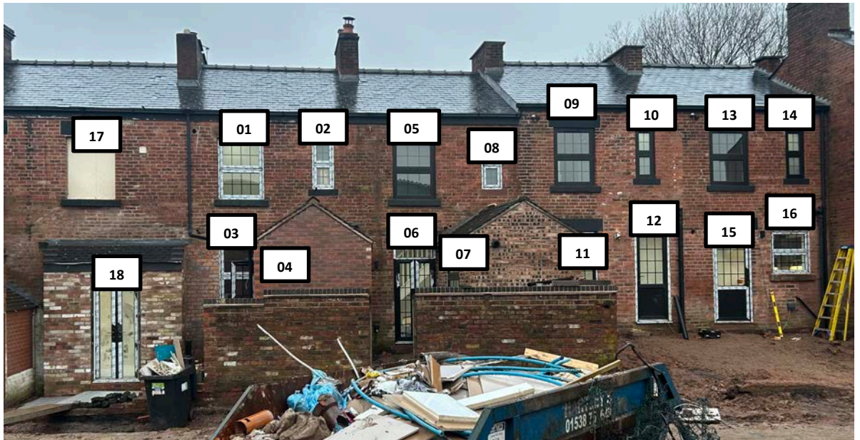
Figure 3: Image of the rear elevation after replacement windows and doors were installed
