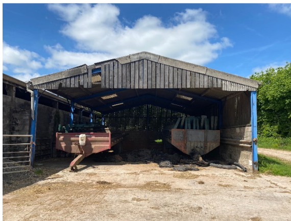
Main Barn – Front Elevation
