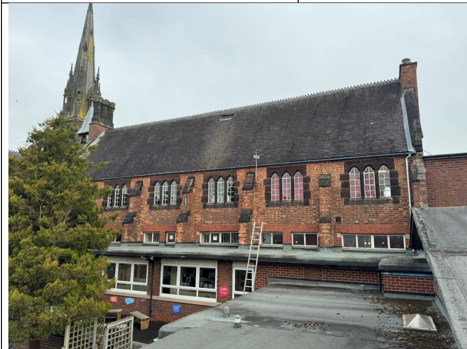
Photograph showing windows and brick surrounds in context to wider historic building.
