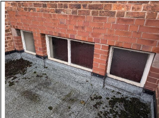
Photograph depicting 'red' brick surround and windows to be removed.
