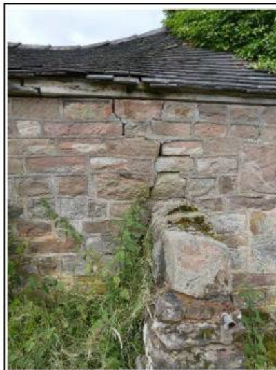
Stonewall at Elevation 3 (Southeast)
