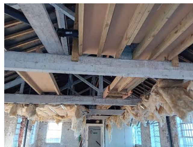
Photo 6: Internal third floor of B1.
