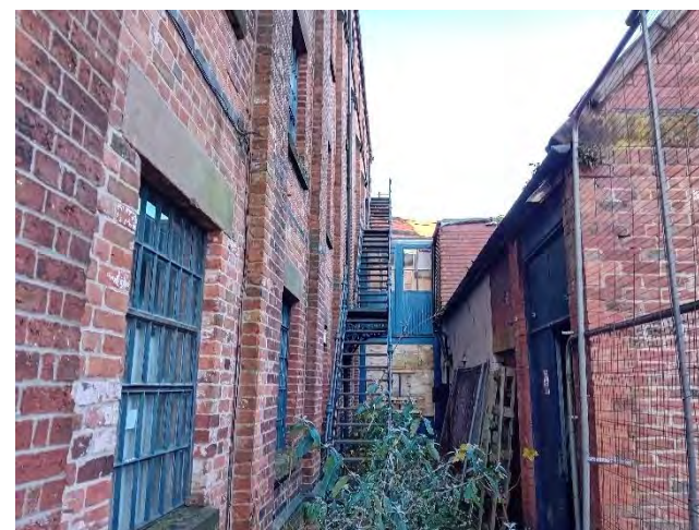
Photo 4: East elevation of B1, west elevation of B2, and the corridor between the two buildings.
