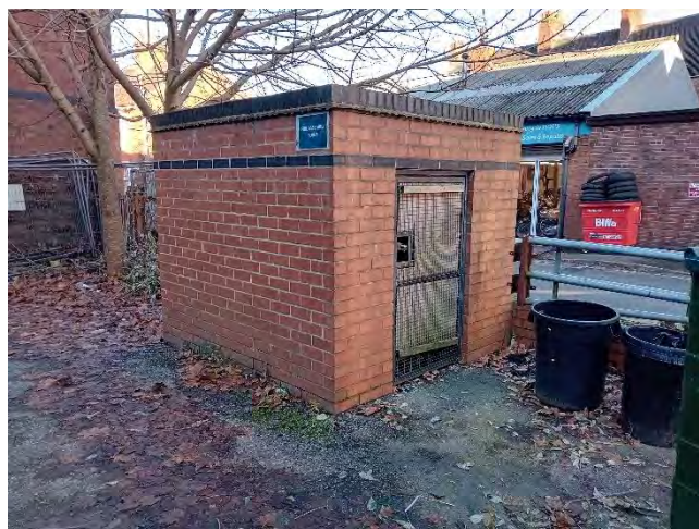
Photo 16: South and west elevations of B3.
