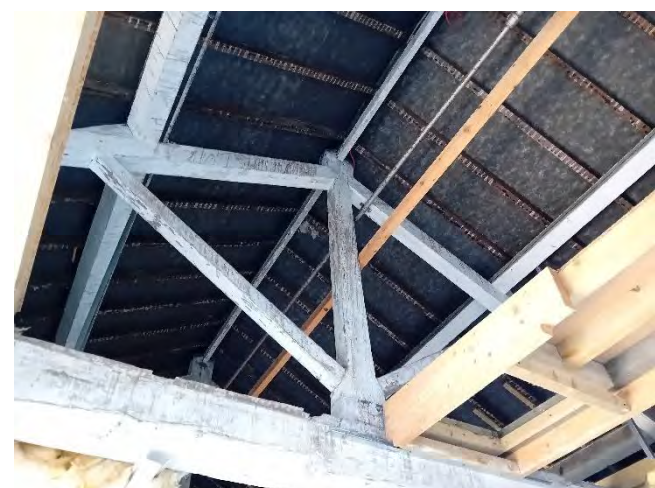
Photo 5: Internal roof structure of B1.
