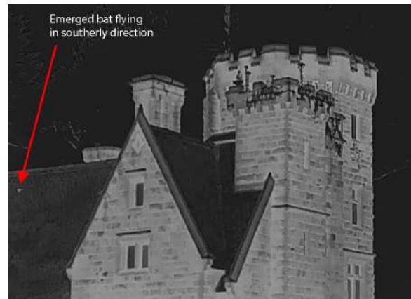
Image 2: common pipistrelle emerging from beneath a tile on the main southwest facing roof pitch of the building
