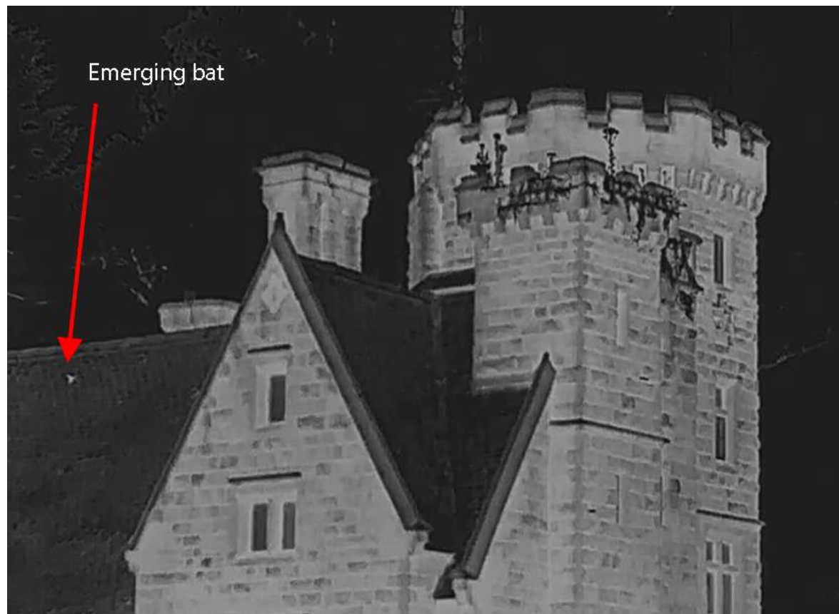
Image 3: another common pipistrelle (in addition to the bat featured in Image 2) emerging from beneath a tile on the main southwest facing roof pitch of the building
