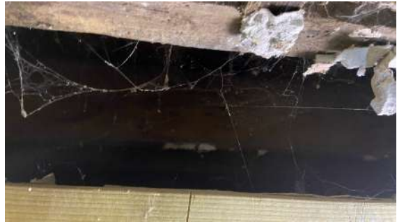
Image 11: narrow loft cavity at northern end of building (viewed from hatch)
