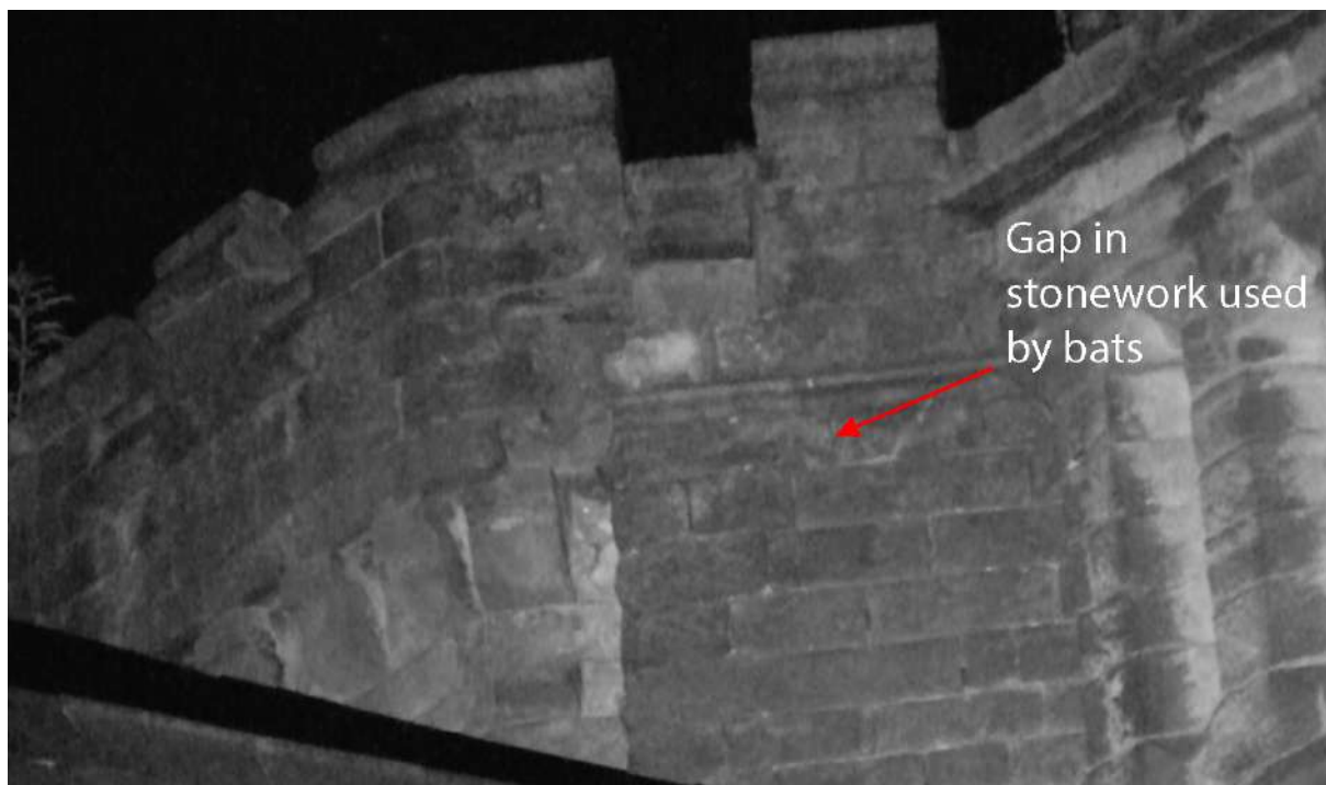
Image 7: red arrow points to area in which access between stonework used by bats is located on eastern side of apse
