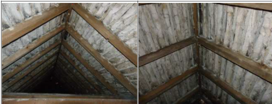
Roof Structure – Ridge Beam, Rafters and Battens
