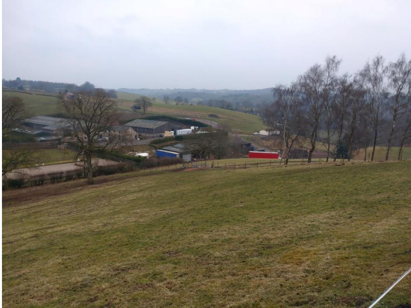
Figure 9: South east of the barn
