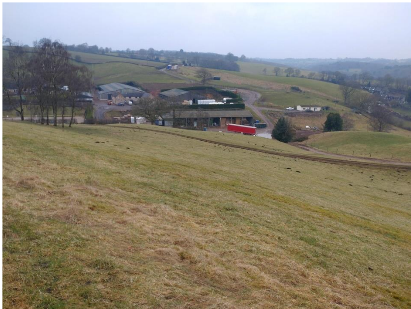
Figure 10: Due east of the barn
