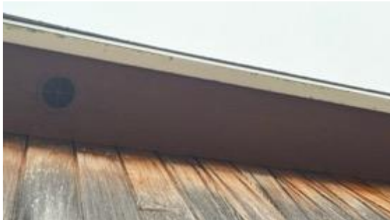
Photo 3: views of the tightly-fitted soffits
