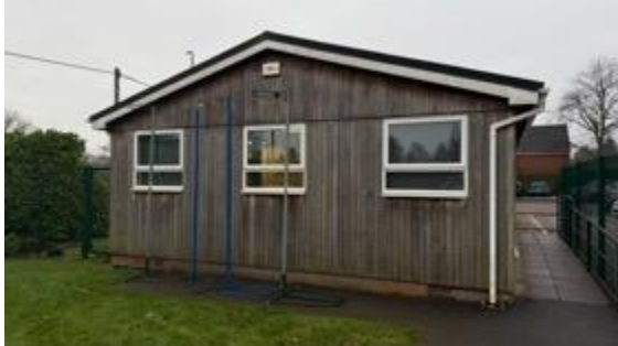
Photo 1: views of the timber-clad gable
