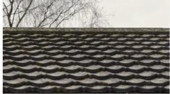
Photo 2: views of the tightly-fitted roof tiles
