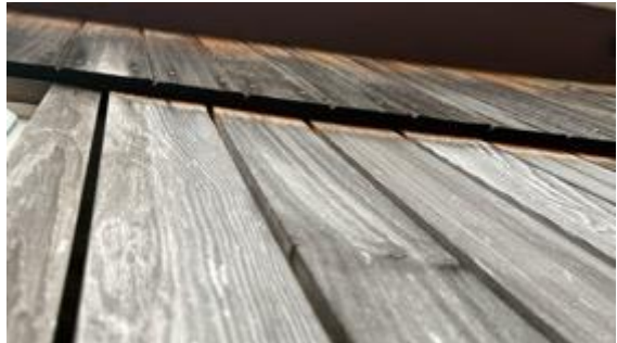
Photo 4: timer cladding fitted to the sides
