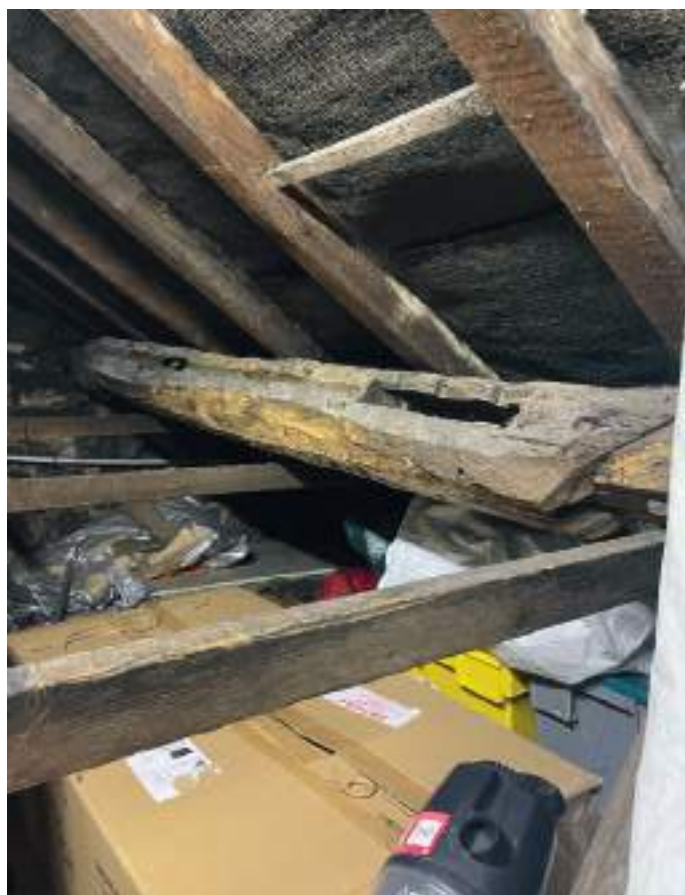
17-19. Roof truss of 17th century origin but re-used on this new alignment in the 19th century, with King post, adapted with the King post cropped at the base and a new tie beam added, along with a pair of raked struts. It is likely that the metal strap was added at the same time to prevent roof spread. Purlins (below) with off-set scarfed and tenoned joints. The purlin to the right is re-used with sockets for additional braces, possibly the remains of a former cruck blade or wall framing. The rafters are all modern (20th century) and the pitch of the roof appears to have been altered during re-roofing, possibly in conjunction with raising the end chimney stack.
