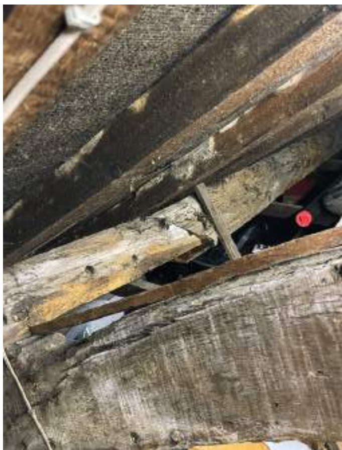
17-19. Roof truss of 17th century origin but re-used on this new alignment in the 19th century, with King post, adapted with the King post cropped at the base and a new tie beam added, along with a pair of raked struts. It is likely that the metal strap was added at the same time to prevent roof spread. Purlins (below) with off-set scarfed and tenoned joints. The purlin to the right is re-used with sockets for additional braces, possibly the remains of a former cruck blade or wall framing. The rafters are all modern (20th century) and the pitch of the roof appears to have been altered during re-roofing, possibly in conjunction with raising the end chimney stack.
