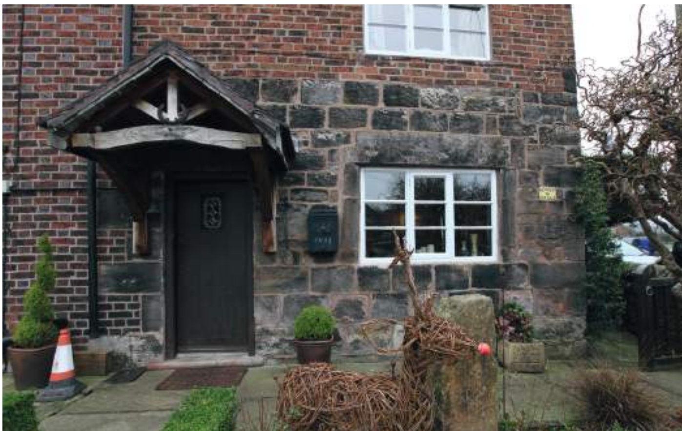
10. 17th century masonry with altered 17th century window. The moulded jambs remain whilst the cill has been lowered and the lintel has been replaced. The door to the left is probably remodelled & extends beyond the line of the straight joint at first floor level.
