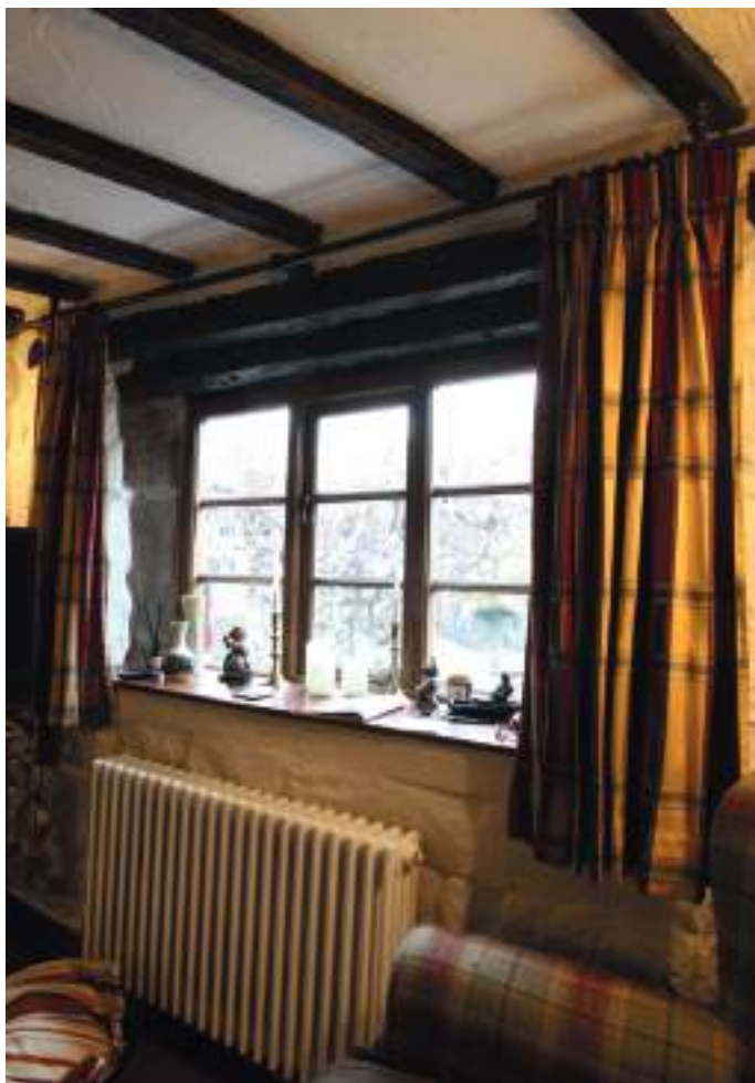
11-12. Two internal views of the altered 17th century window, with oak internal lintels.
