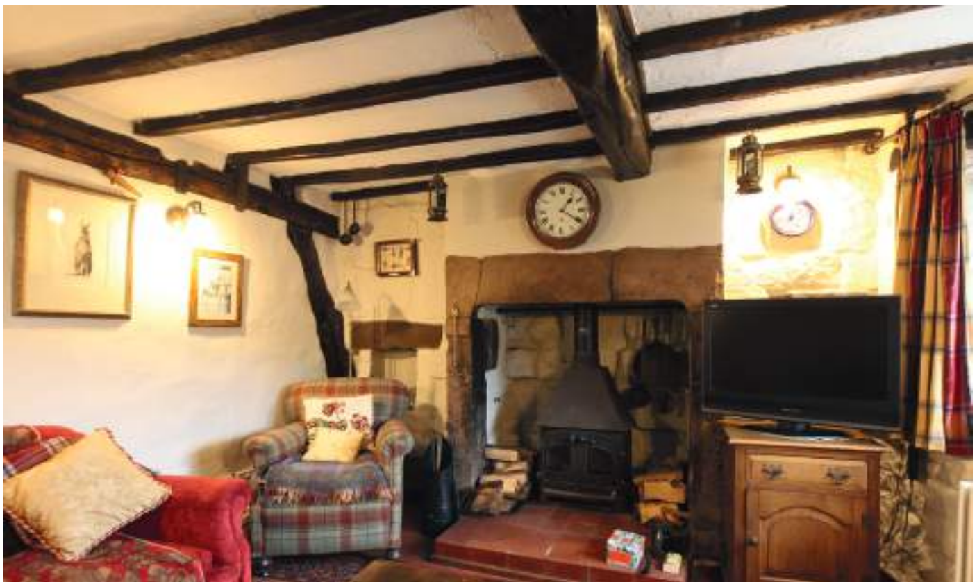
22. Lounge - view looking towards the hearth and the road. The massive spine beam appears to be 17th century but has been de-frased and any signs of adzed chamfers have been removed. The joists are later. The fireplace surround is simple with subtle blocking. The style of lintel with a depressed arch is found in the 17th century but the lack of any mouldings and the smooth face of the lintel and blocking to the jambs suggests it has been re-dressed.
