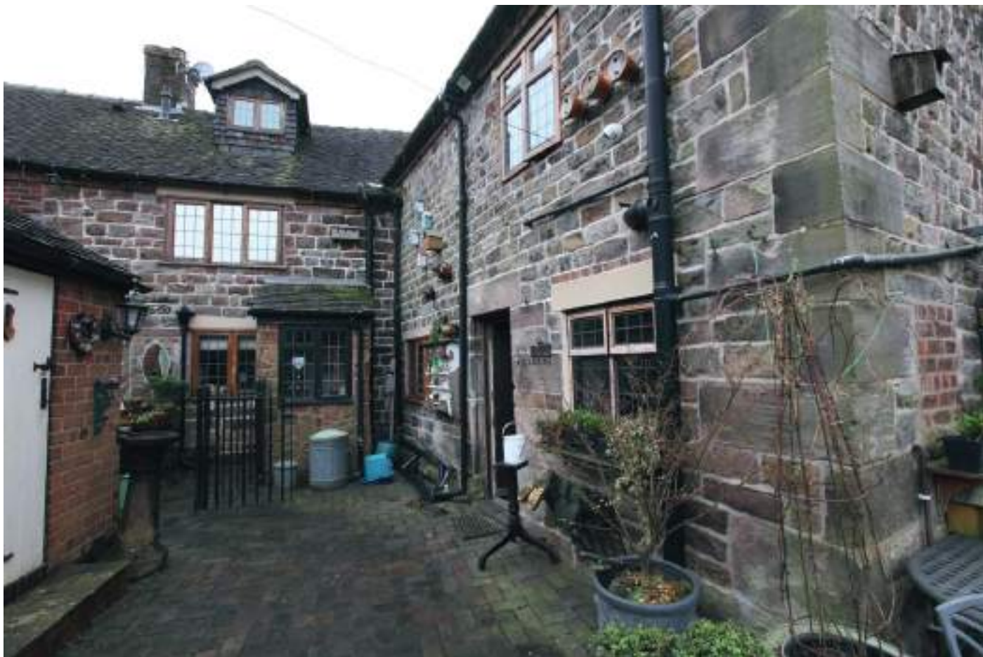
5. Rear elevation of Brook Cottage and Middle Cottage to the left. The stone masonry walls seen here of Middle Cottage were originally part of the same L-plan building, as depicted on the 1882 OS map. The stone masonry is very evenly coursed and this may represent a remodelling, as there is no evidence that the 17th century masonry continued to the corner quoins. Instead, the 17th century masonry terminated at the stone plinth or the doorway. All three windows on this rear elevation are modern (mid-late 20th century) with concrete lintels.
