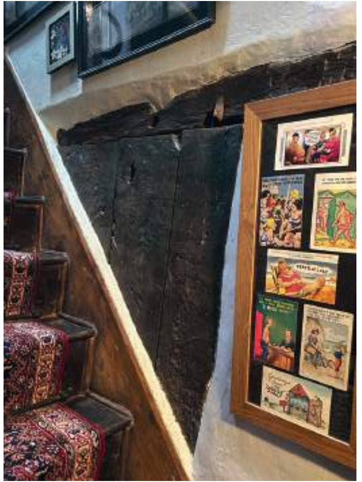
20 - above left. The soffit of the principal rafters to the truss have a 19th century oak strut. The two sockets on the underside are the remains of the mortices for two arched braces. Each of these was secured with oak pegs - peg holes can still be seen. 21 - above right - remains of oak boarding to the staircase wall and oak lintel with pegholes. The function of this boarding is obscure.
