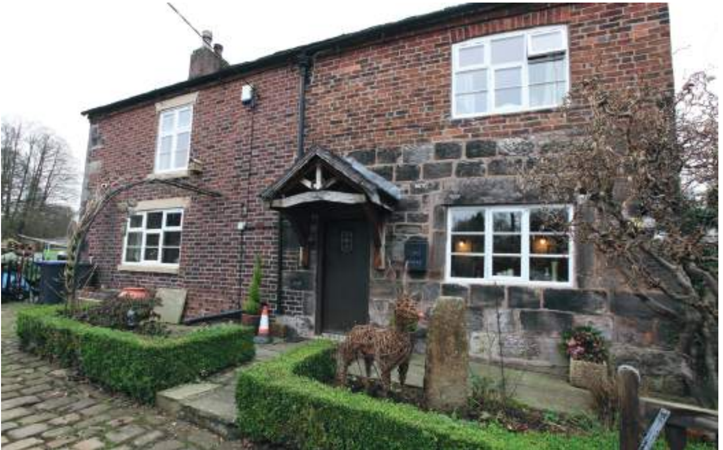
3. Elevation to the south overlooking the brook. Three distinct phases are represented in this elevation although the window pattern is unifying, as is the patina of mellow brick and stone. The first floor window to the right has a shallow segmental arch, also known as a cambered brick arch (comprising a square top and curved bottom), which is found typically during the first half of the 18th century. The eaves to this elevation is plain corbelled and of two clear phases.
