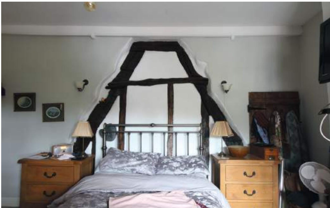
15, First floor - upper part of the cruck frame on the internal wall. This reveals that the dwelling was remodelled with a higher eaves to create a taller two-storey dwelling. The setting out of the timber studwork may represent the location of a first floor doorway. Spurs are visible at roughly the mid-point of each brace, which would reflect the original eaves level.
