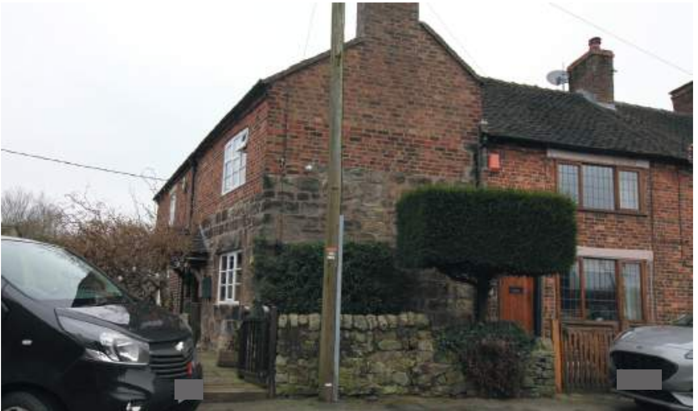
2. Gable end to the street, with 17th century stone masonry, area of remodelled brickwork to the gable incorporating two phases of brickwork, the later phase a significantly paler colour.
