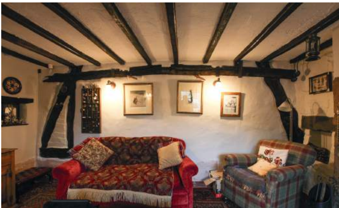
16. Lounge with lower part of cruck. The girding beam reveals the original ceiling height of the 16th century dwelling, which is not dissimilar to the current ceiling height, although these joists are probably 19th century. The alignment of the original three beams which ran across the girding beam is represented by the three sockets in the upper face of the girding beam. Whether this is the closed truss or an internal truss is unclear. If it was an internal truss the remaining 16th century bay was demolished in the 17th century and the 'wing' was aligned perpendicular to the 16th century range.
