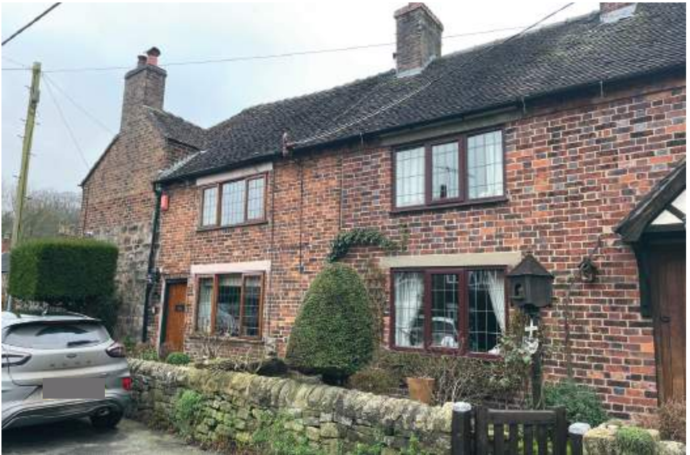
1. Elevation of Middle Cottage and Yew Tree Cottage. These both share a sawtooth eaves which is very typical of the 18th century. Map regression indicates that Middle Cottage was once part of Brook Cottage. Windows and doors to both cottages have been remodelled. There is a straight joint between Middle Cottage and Yew Tree Cottage, which also has flared headers typical of the early 19th century. It is likely that a further cruck truss was originally located on the line of this straight joint.
