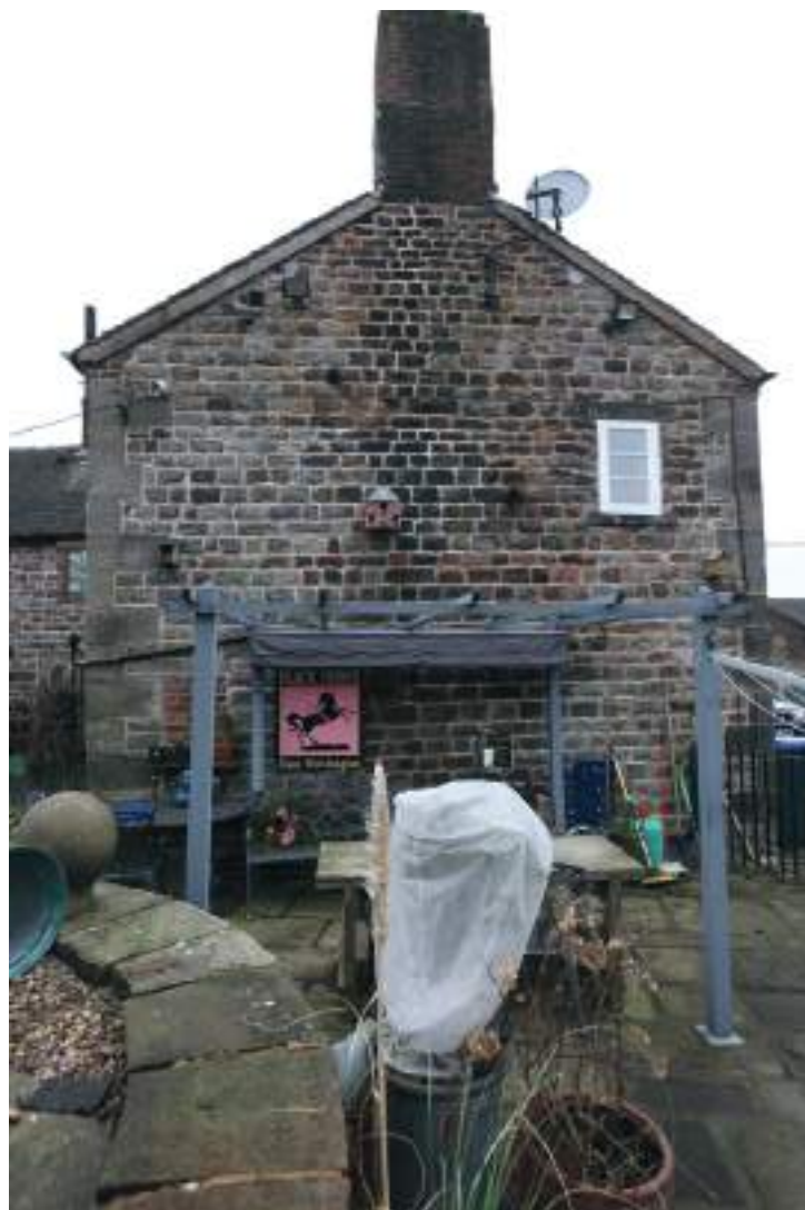
5. Rear elevation of Brook Cottage and Middle Cottage to the left. The stone masonry walls seen here of Middle Cottage were originally part of the same L-plan building, as depicted on the 1882 OS map. The stone masonry is very evenly coursed and this may represent a remodelling, as there is no evidence that the 17th century masonry continued to the corner quoins. Instead, the 17th century masonry terminated at the stone plinth or the doorway. All three windows on this rear elevation are modern (mid-late 20th century) with concrete lintels.
