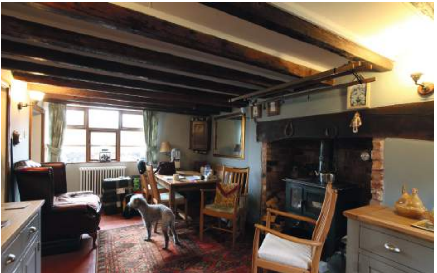
14. Dining Room to the 19th century bay. The hearth and timber lintel are modern and are a remodelling of a smaller hearth. The ceiling joists are pitch pine and 19th century.
