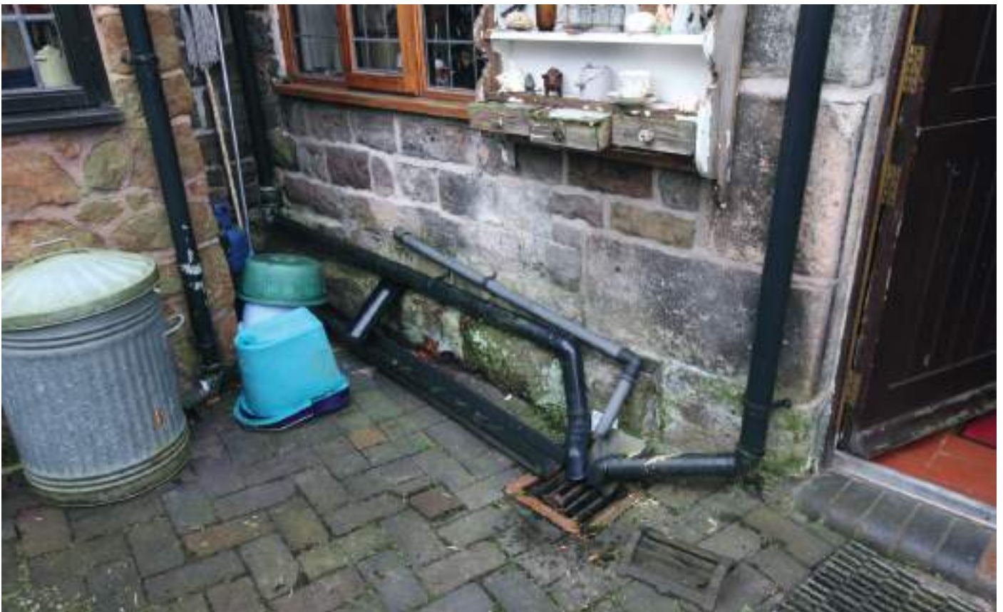
4. Rear elevation with remains of a 17th century stone plinth. This demonstrates that the 17th century building extended as far as the back door before it was extended in the 19th century, so there is a degree of overlap in the front elevation masonry phasing.
