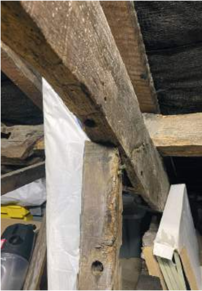
20 - above left. The soffit of the principal rafters to the truss have a 19th century oak strut. The two sockets on the underside are the remains of the mortices for two arched braces. Each of these was secured with oak pegs - peg holes can still be seen. 21 - above right - remains of oak boarding to the staircase wall and oak lintel with pegholes. The function of this boarding is obscure.
