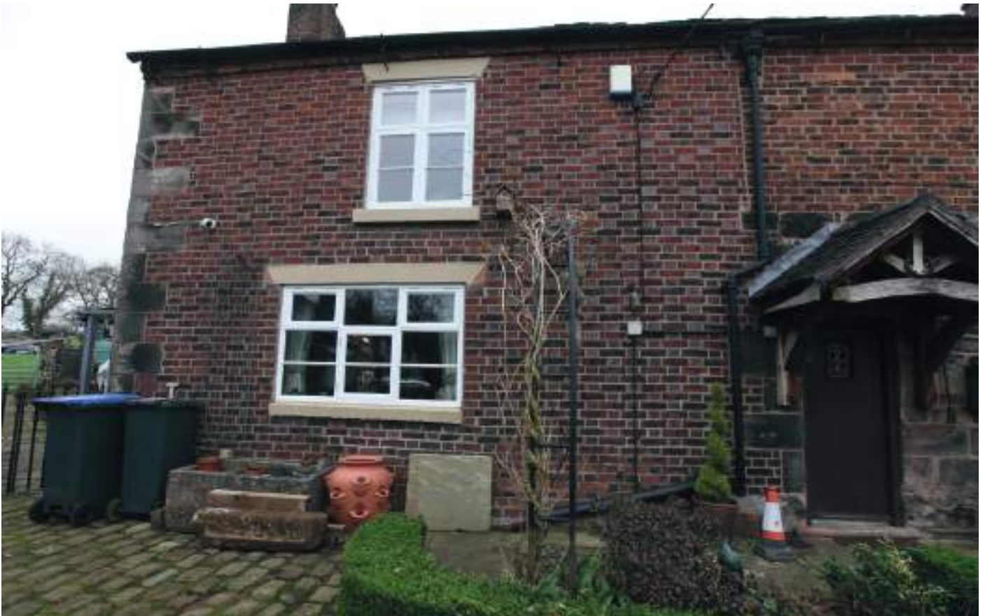
13. Early 19th century Flemish bond brick brickwork and bay extension. The flared headers are a distinct blue colour. The ground floor window has been widened and the lintel appears to be concrete. Original wedge stone lintel to the first floor. A sash window may have been removed and replaced with casements. The distribution of windows is odd because there are no brick closers, which would be expected in conjunction with Flemish bond brickwork, and the right jamb of the first floor and ground floor windows are not directly aligned.
