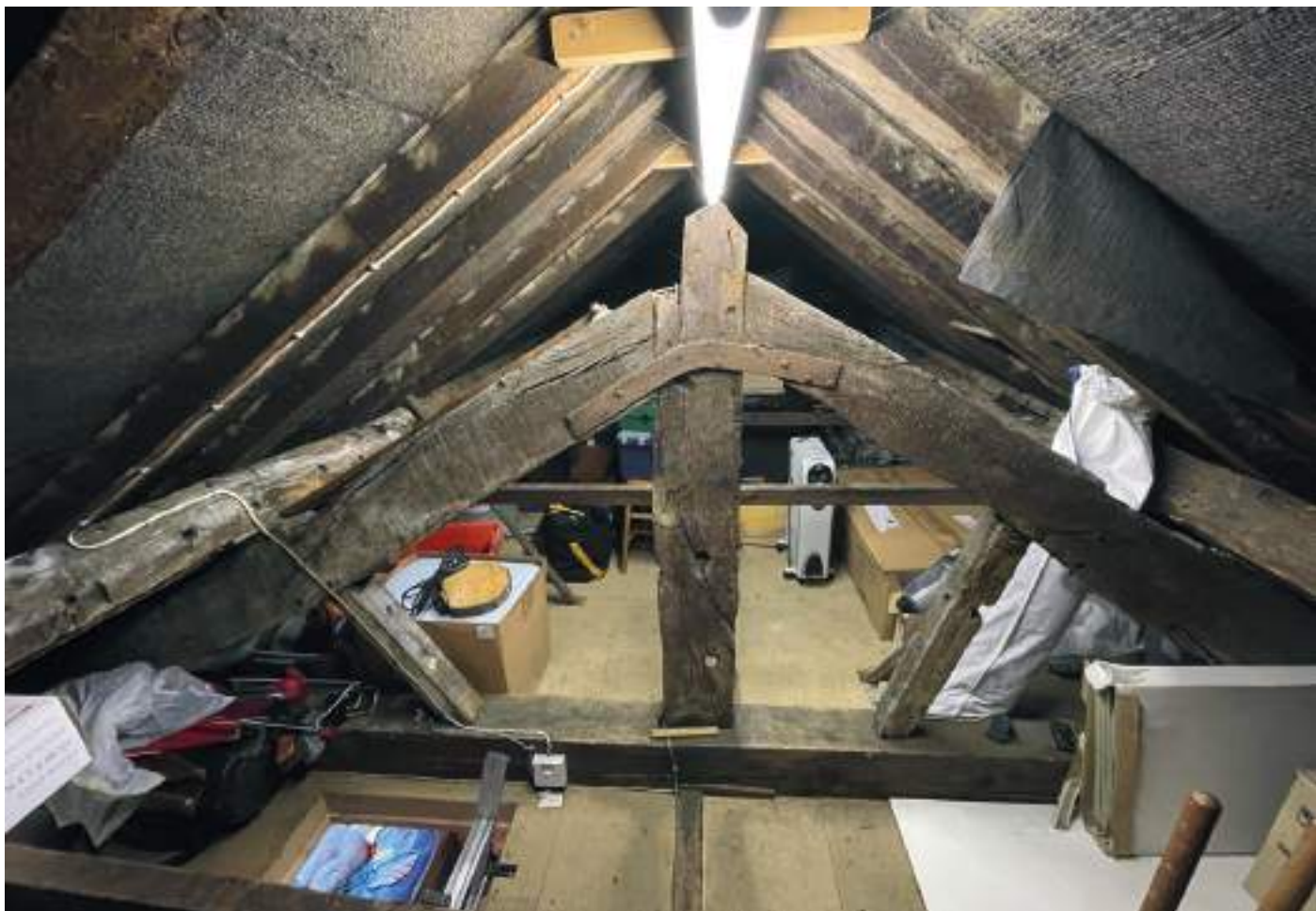
17-19. Roof truss of 17th century origin but re-used on this new alignment in the 19th century, with King post, adapted with the King post cropped at the base and a new tie beam added, along with a pair of raked struts. It is likely that the metal strap was added at the same time to prevent roof spread. Purlins (below) with off-set scarfed and tenoned joints. The purlin to the right is re-used with sockets for additional braces, possibly the remains of a former cruck blade or wall framing. The rafters are all modern (20th century) and the pitch of the roof appears to have been altered during re-roofing, possibly in conjunction with raising the end chimney stack.
