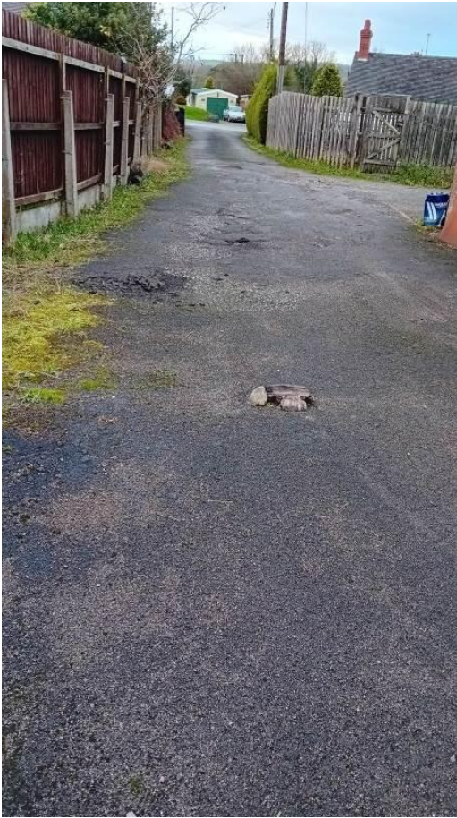
Plate 8: Existing tarmac driveway
