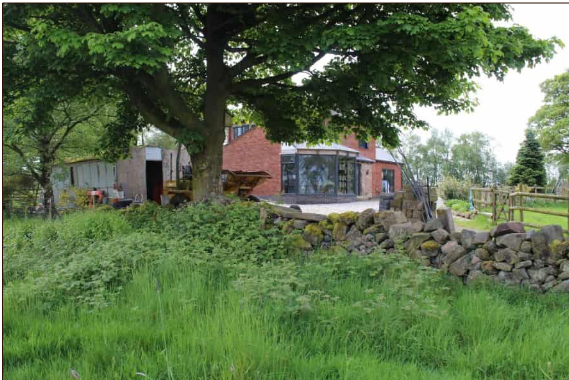
Photo 11: Looking north from within the Site towards new dwelling in the former location of Little Armshead Farmhouse (MST21899)
