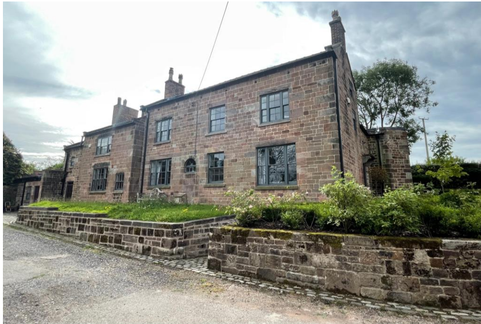
Fig. 4: The north face with a series of later extensions to the left. The extension which is farthest left, now housing a utility room, replaces the pig-sty still present in 1925; Source: ctd architects, 2025
