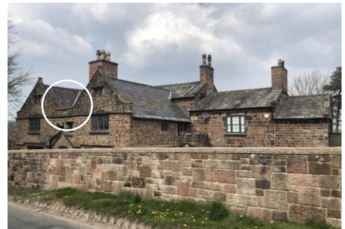
Fig. 3: The south face of the 17 th century range, and right, the west face showing the junction of the two main phases- 17 th century and 19 th century; Source: ctd architects 2021
