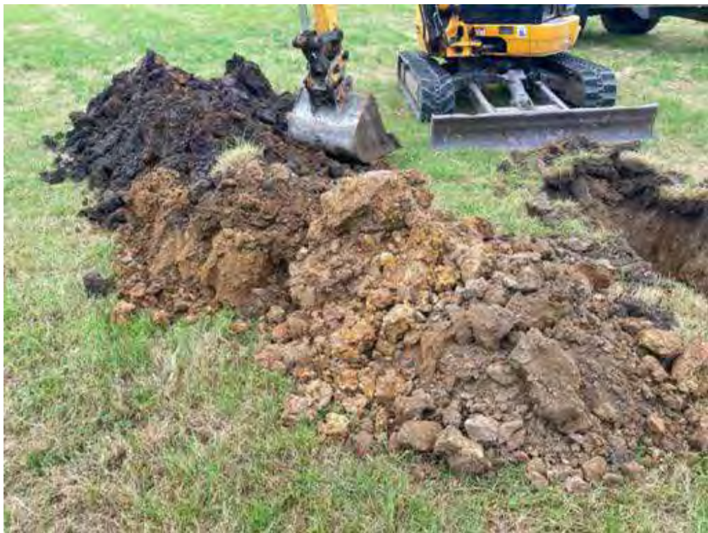
Photograph 12 Description: Spoil excavated from TP01 Date: 20/07/2022
