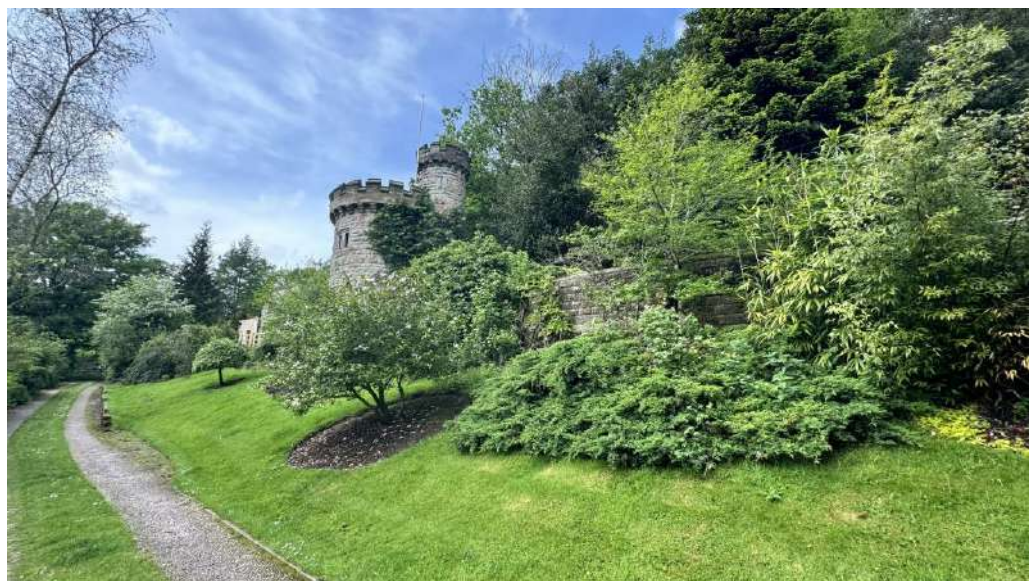
Fig.1 Folly Tower from the east, with Rock Cottage just visible in the background, 2015 (source: ctd architects)
