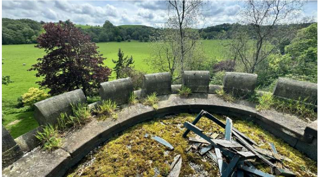
Fig.7 Existing roof and crenellated embattled parapet (source: ctd architects)
