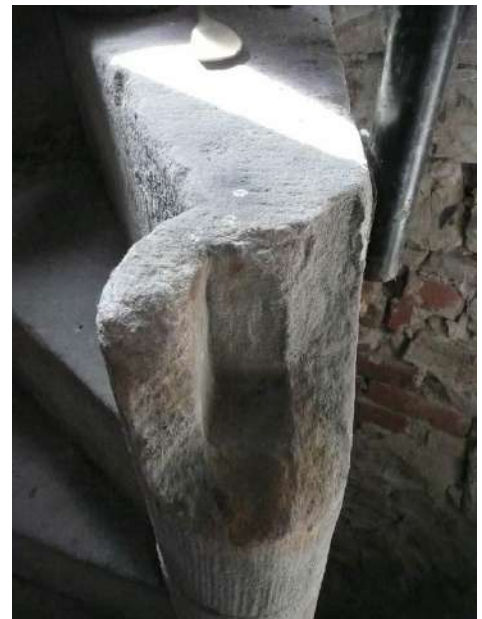
Fig.10 (left) & Fig. 11 (right) Existing defective 'modern' timber windows to be replaced with new metal casements (left) and (right) location of proposed stone indent repair to the top of the stone spiral staircase central newel post (source: ctd architects)
