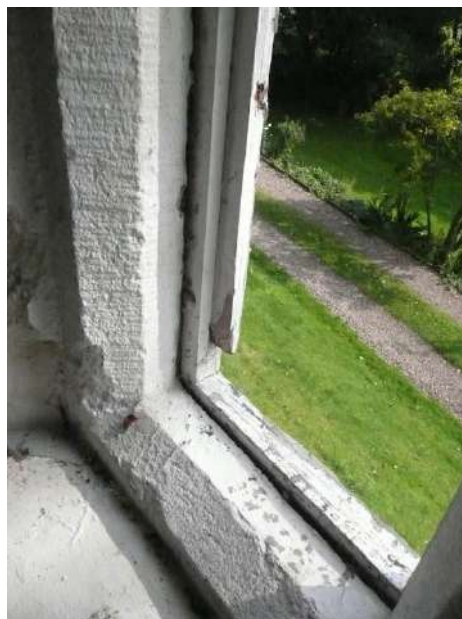
Fig.10 (left) & Fig. 11 (right) Existing defective 'modern' timber windows to be replaced with new metal casements (left) and (right) location of proposed stone indent repair to the top of the stone spiral staircase central newel post (source: ctd architects)
