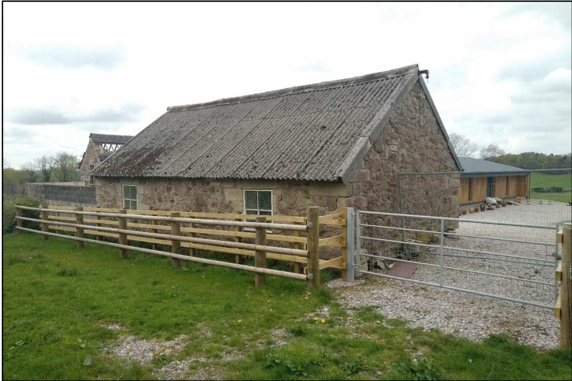
Figure 2: Rear elevation of the standstone barn
