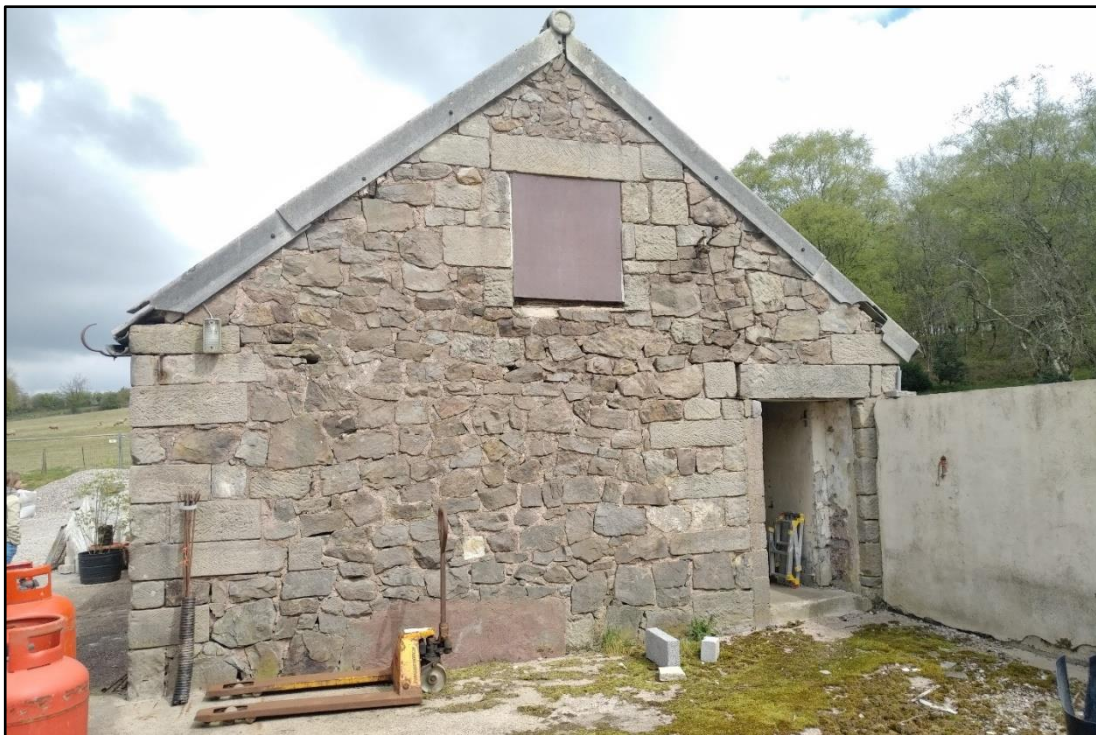
Figure 5: Gable end of the stone barn
