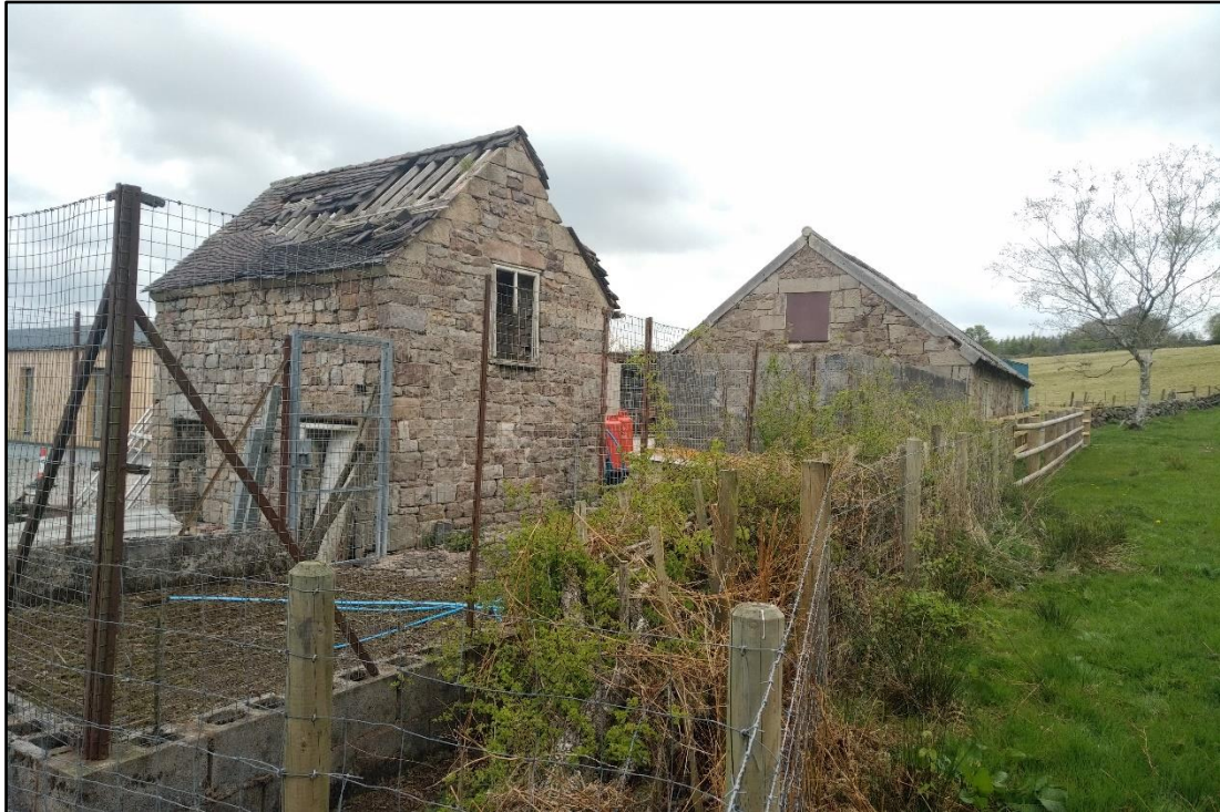
Figure 4: South elevation of the stone barn and the outbuilding in the foreground
