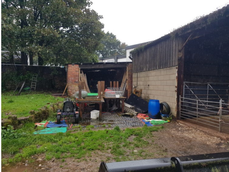
Photo - see structure to be demolished and adjacent barn
