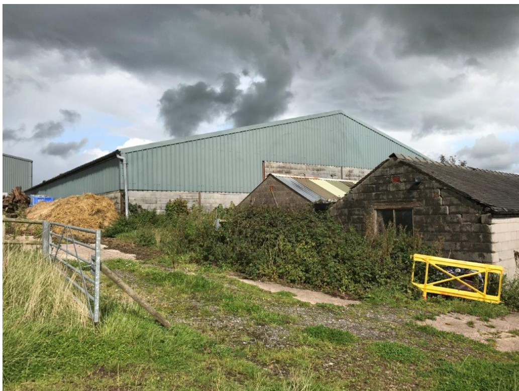
Large agricultural portal frame buildings dominate the land to the north-west of the farm group over the brow of the rising land.
