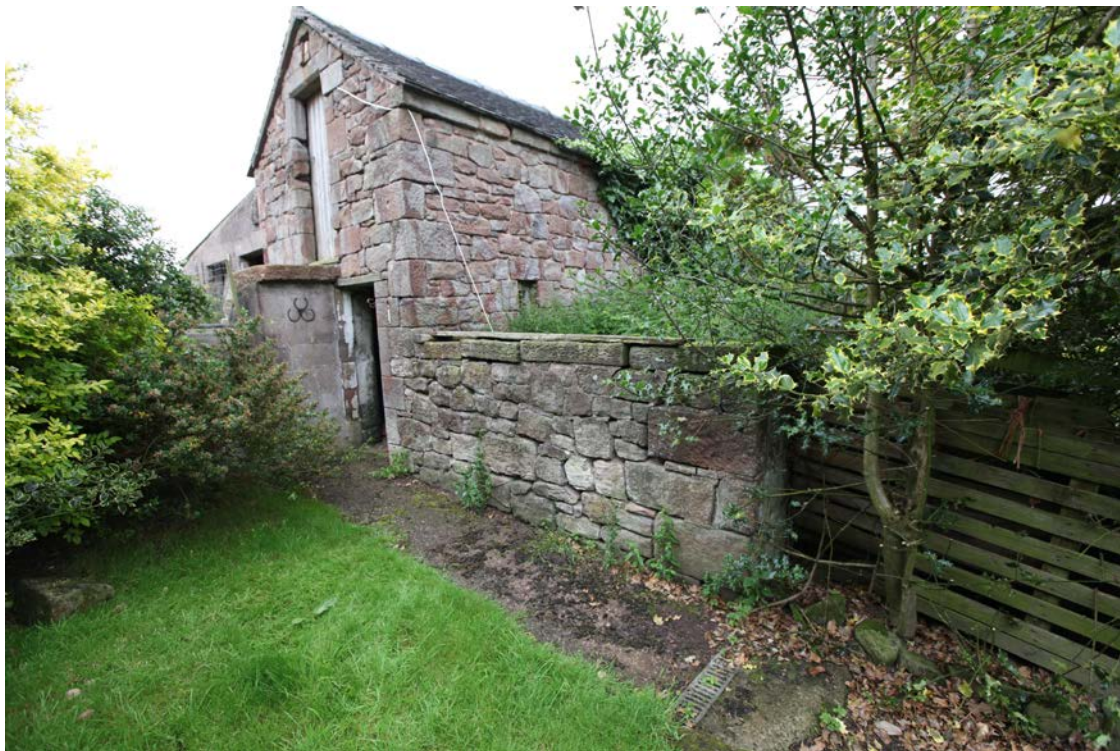
Combination building of pigsties, hayloft and privy – probably mid 19 th century
