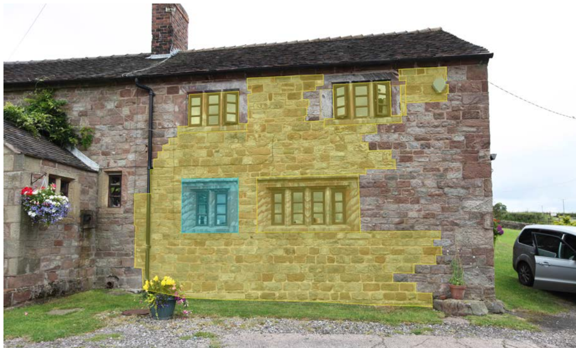
Area of reconstructed stonework, approved in 1992 – eastern bay. The 'blue' window is a new mullioned window approved in 1992
