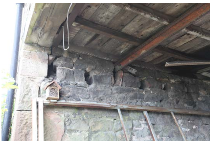
Inserted and raised floor into cart bay with altered joists and lintel. The original sockets for the joists which ran axially are still visible.
