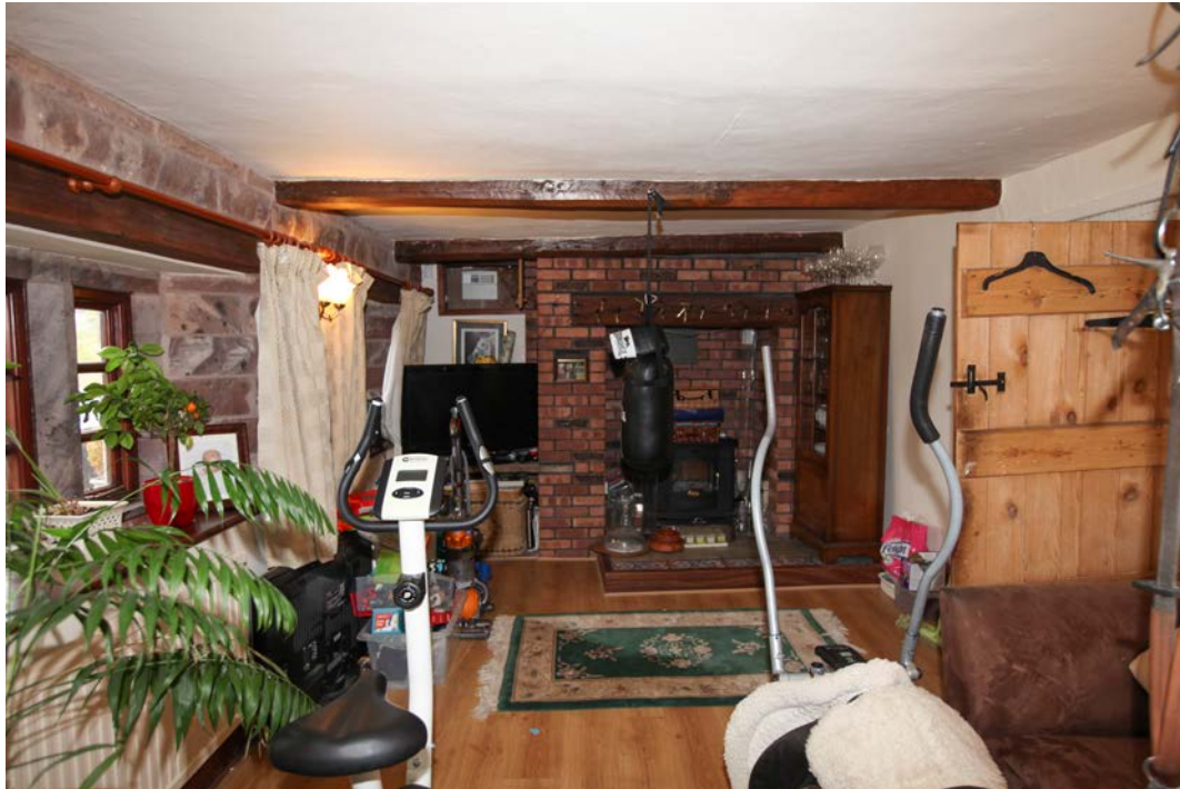
Former smokehood with its bressumer is visible with a modern brick chimney breast inserted. The window wall to the front of the house has been rebuilt although transverse beams appear to be in-situ.
