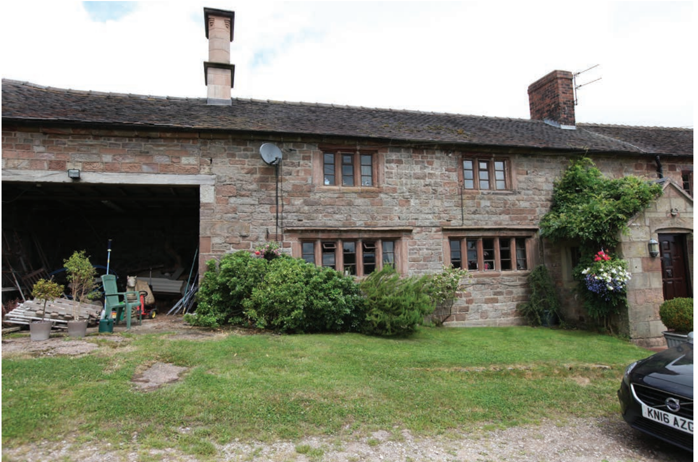
Pl. 3 View of the south-facing elevation. The modern porch of 1984 covers the original entrance doorway into the Houseplace or Hall. The open cartshed to the left is a later 19th century alteration and may relate to the documented presence of a 'carter' at Rownall in the 1861 and 1871 census returns.
