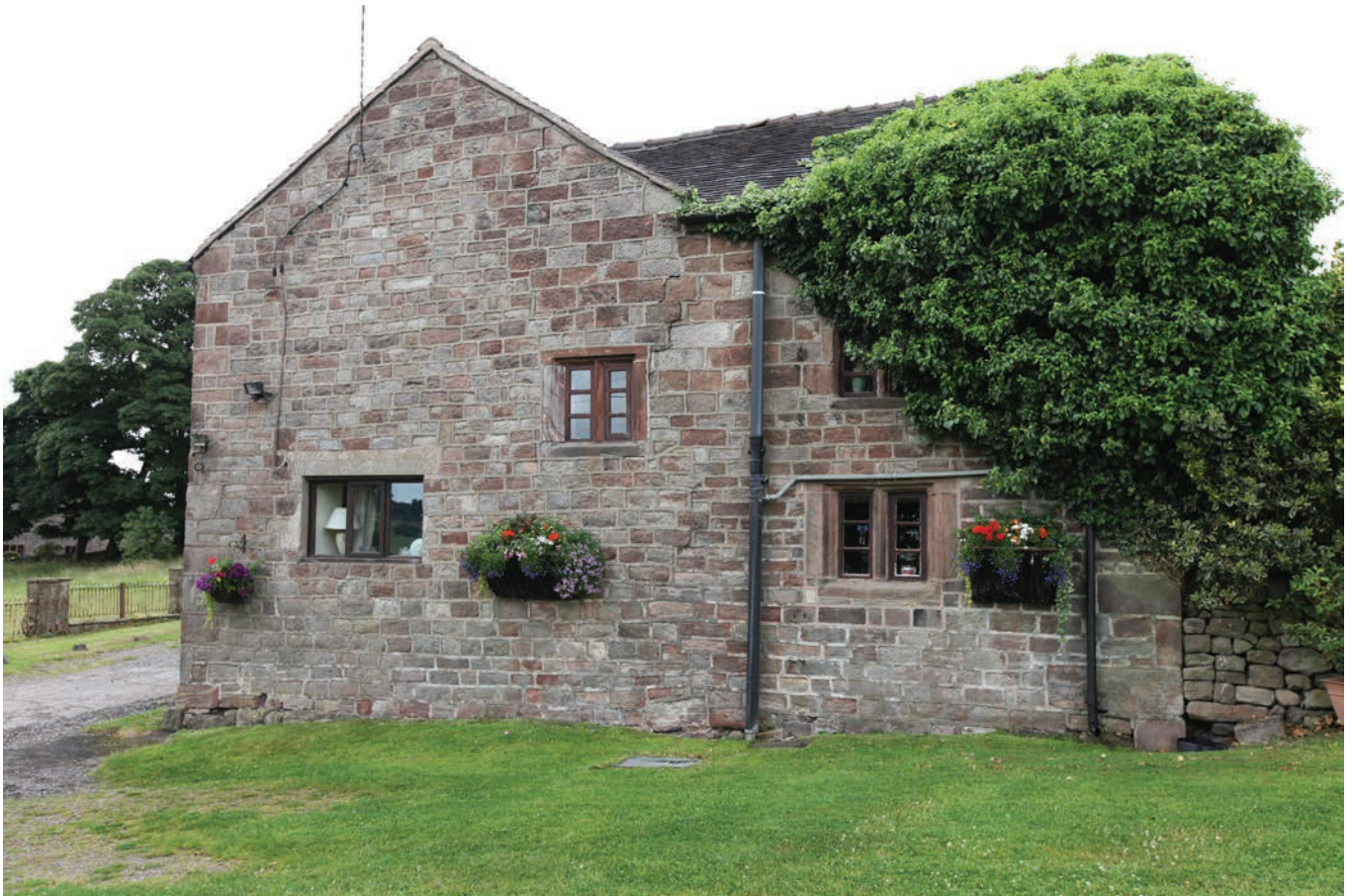
Pl. 7 Eastern gable end. This elevation has undergone considerable alteration. The larger masonry courses towards the gable suggest a large area of reconstruction, possibly undertaken in the 18th century. The original stone coped gable has also been removed. There are indications that this part of the building may have originally been a single-storey kitchen wing using the earlier cruck trussed frame, which would account for the change in masonry. When it was altered in the later 17th century and raised to two storeys, a staircase window was inserted.
