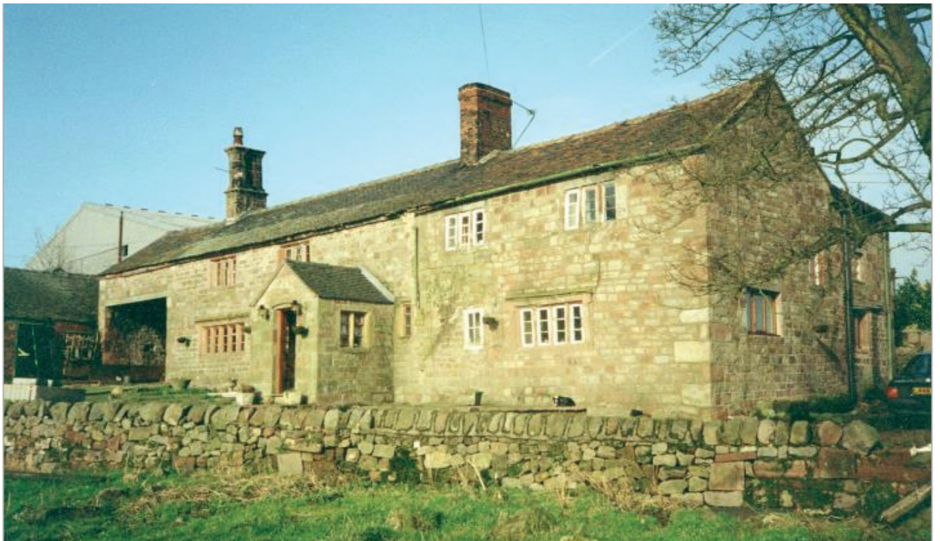
Pl. 4 Photograph of the entire south-facing elevation taken circa 1984 prior to alterations.
