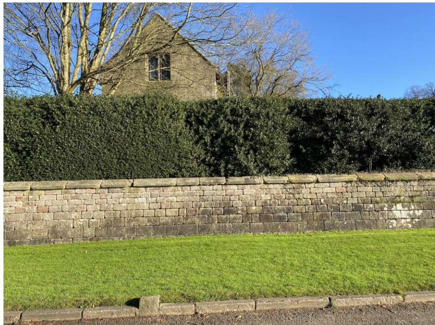
Fig 10. The western boundary wall showing the west gable elevation of the Coach House, ctd architects 2024
