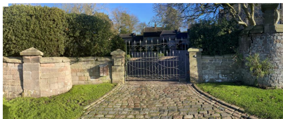
Fig 7. The western boundary with existing vehicular entrance to Tollgate Road, 2024
