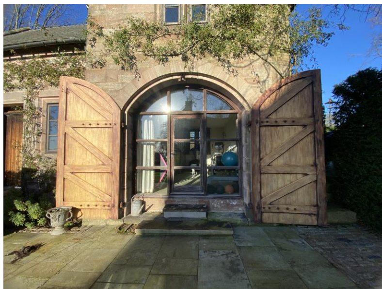
Fig 6. View of the South elevation of the Coach House showing the former cart entrance infilled with window and glazed door, 2024
