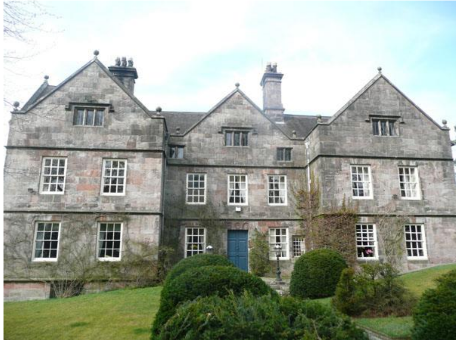
Fig 5. View of the South front elevation taken from the separately listed gates and railings at the boundary with Heath House Lane, 2014
