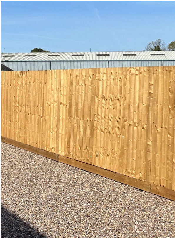
Timber Close board fence
