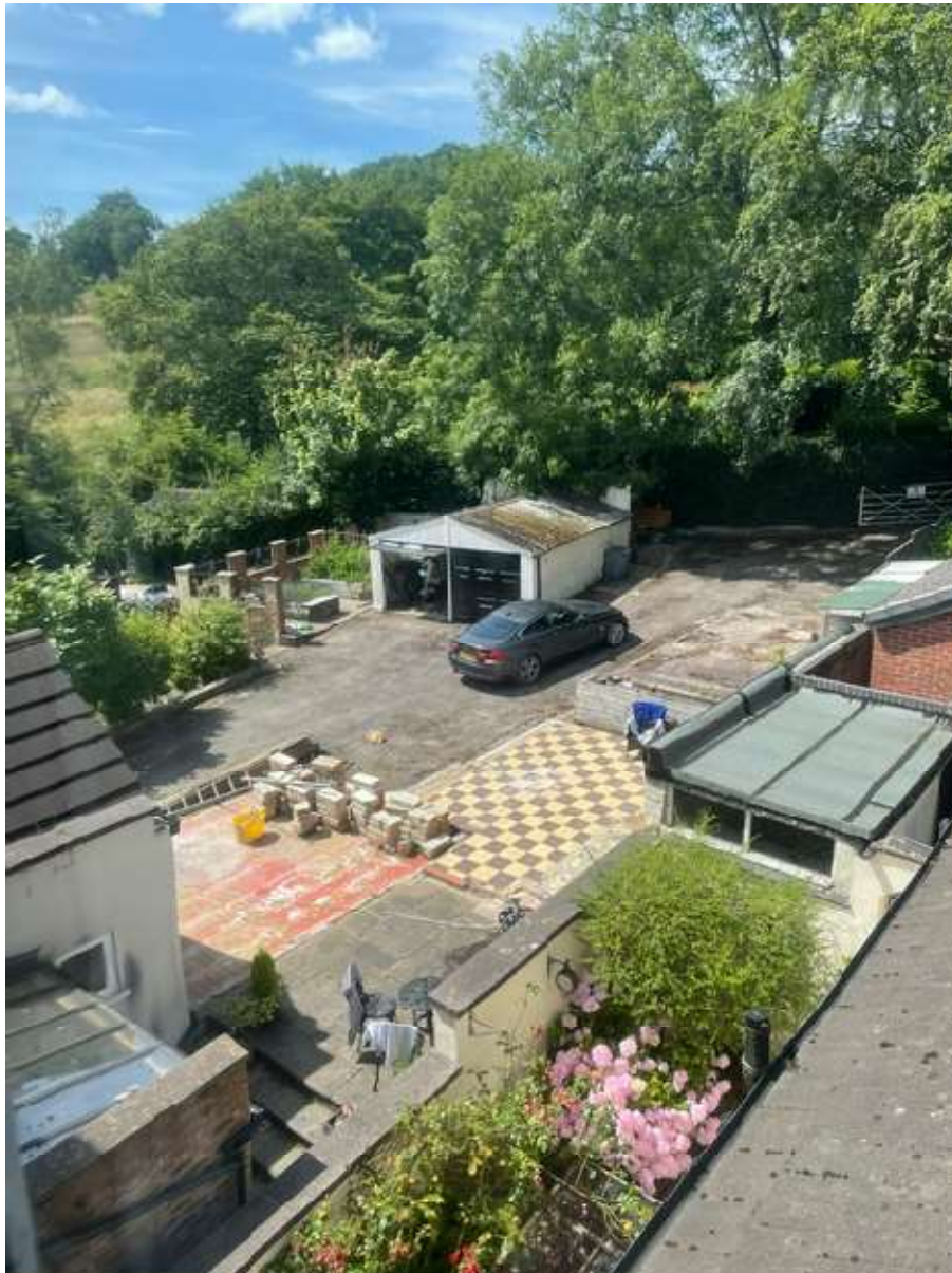
Photo showing the footprint of the part extension that was demolished and our backyard and roof of our house on the bottom right corner– the proposed extension would be closer to our house and the footprint of the demolished extension
