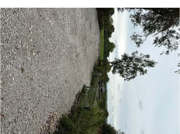
figure 1: Surface upgraded with MOT hardcore
