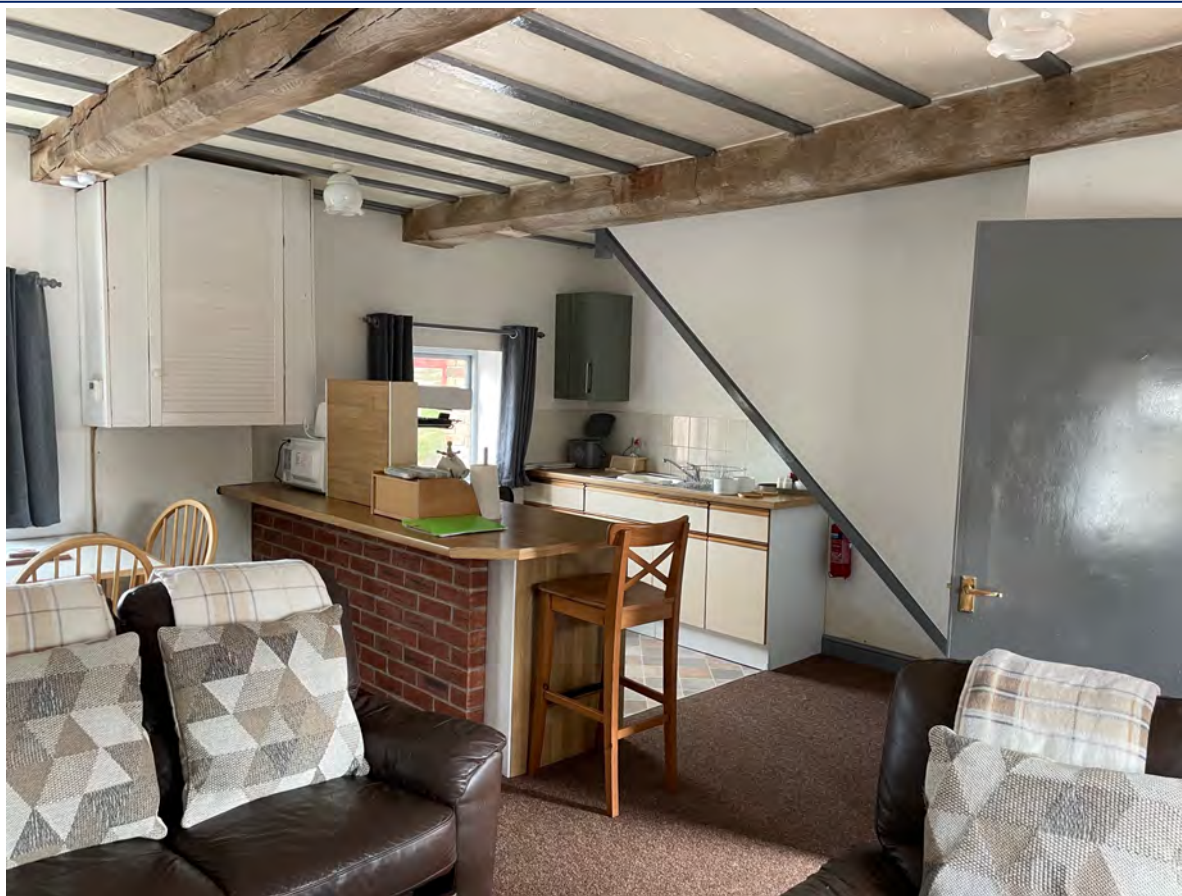
Plate 10. Example of retained original chamfered spine beams with carved stops.
