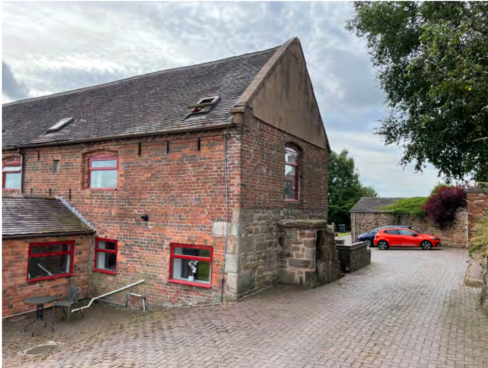
Plate 8. Western gable end of the northern range with stone steps and dog kennel beneath.
