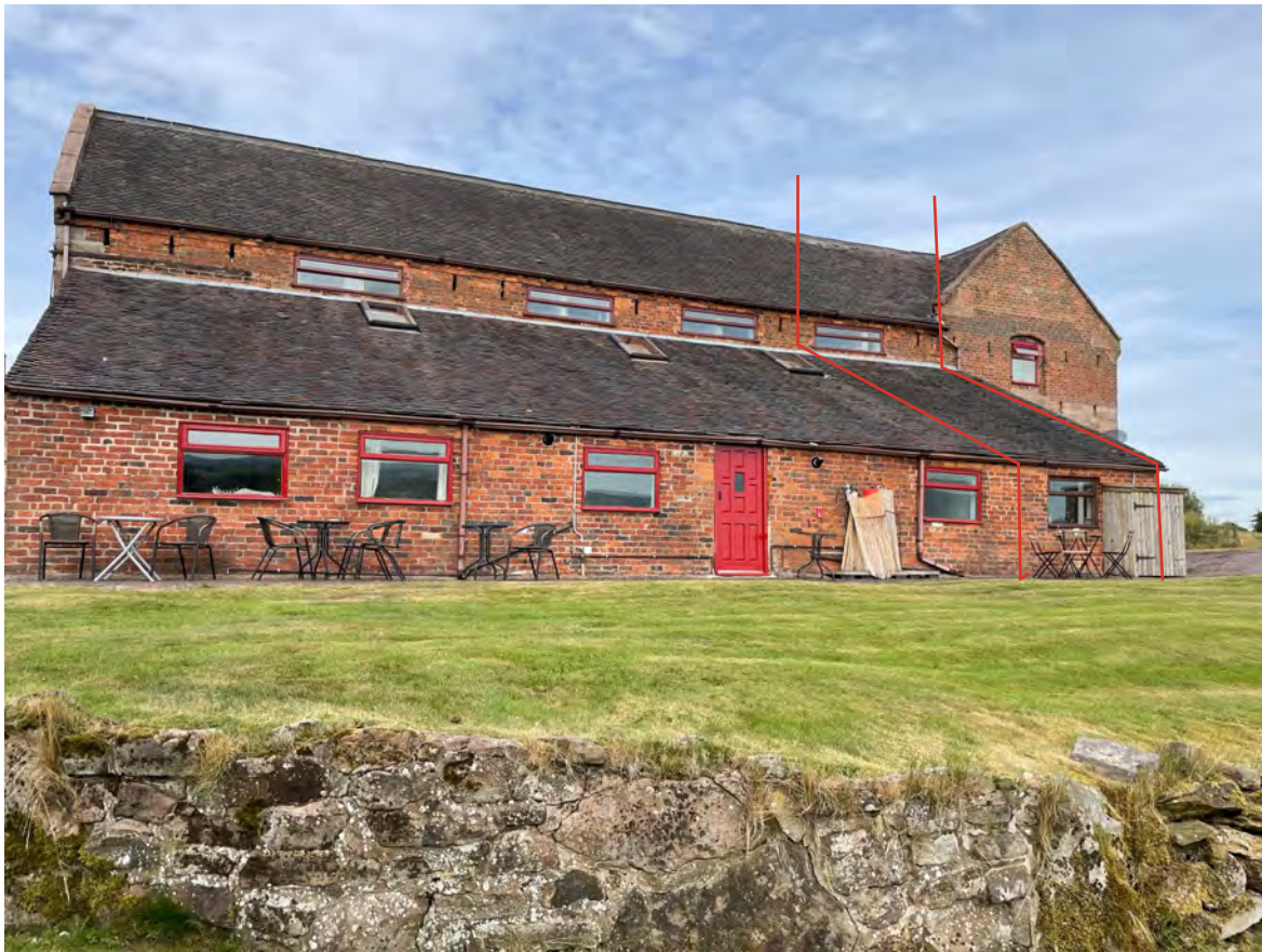
Plate 6. Eastern elevation of the barn showing later adjoining lean-to.
