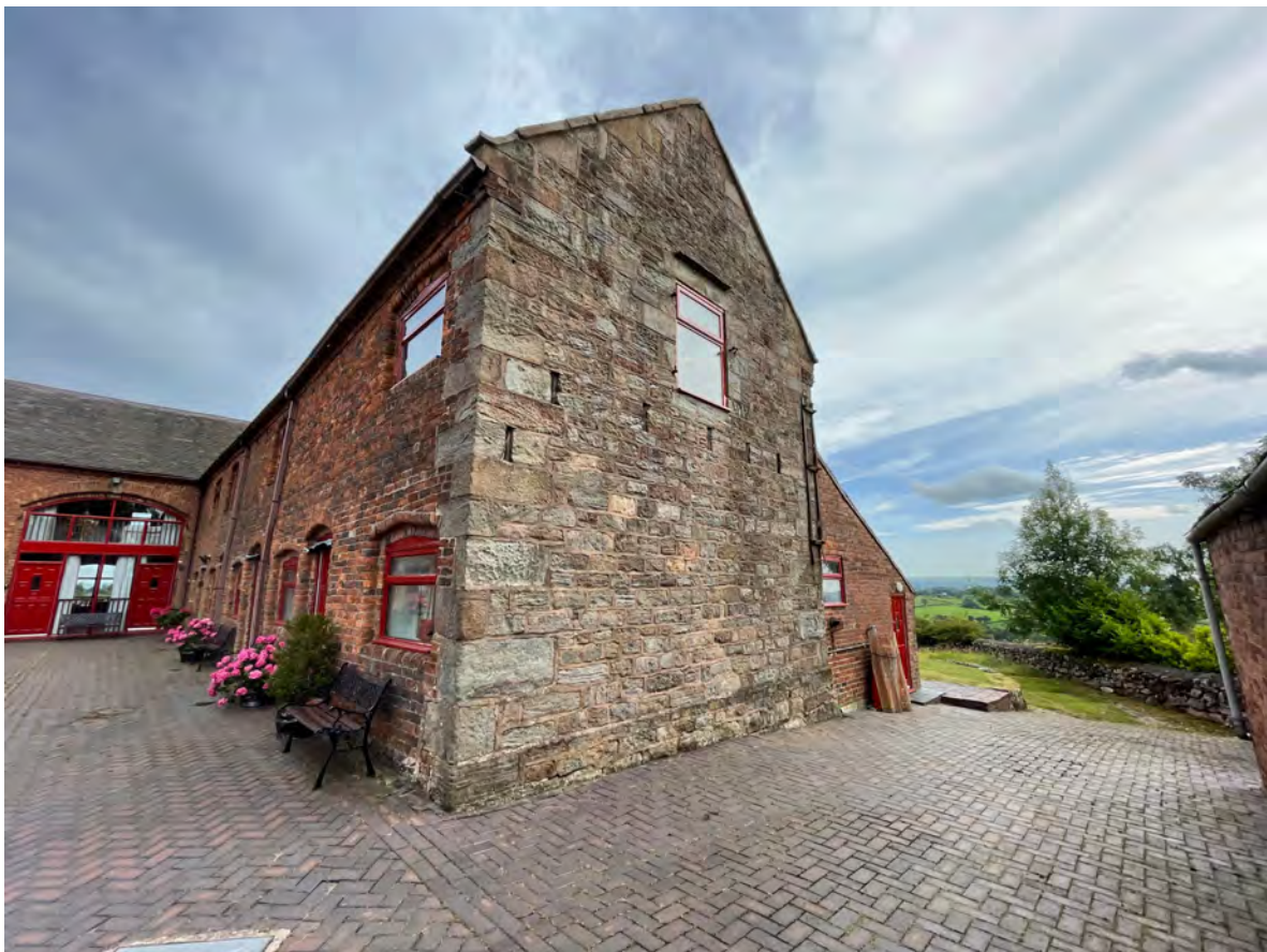
Plate 7. Southern gable end of the eastern range of the barn.
