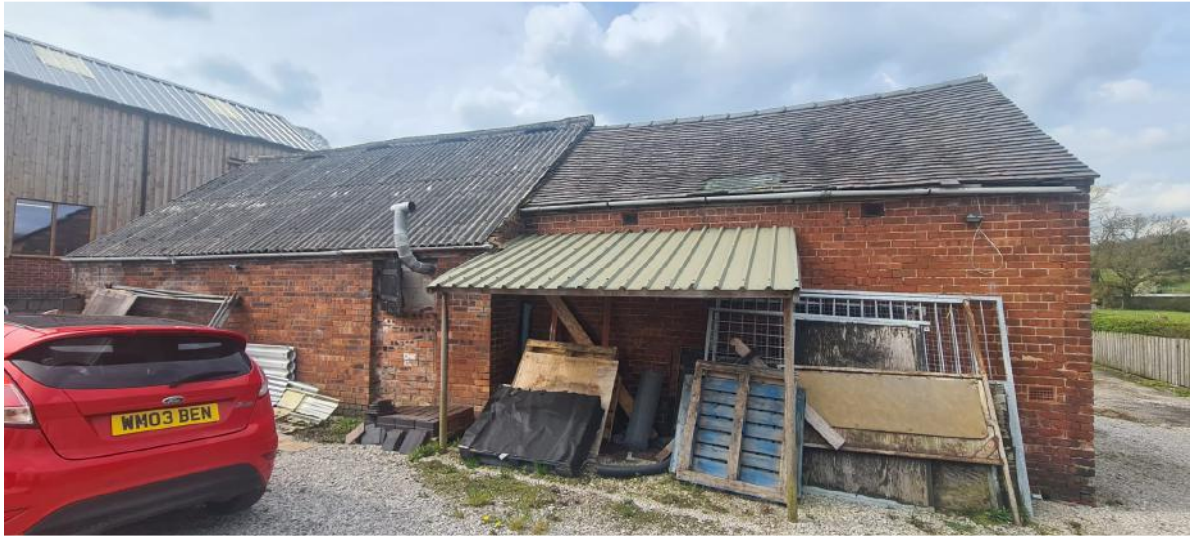
Fig 13. Rear elevation. Doorway partly blocked up with bowed wall panel where lean to is.
