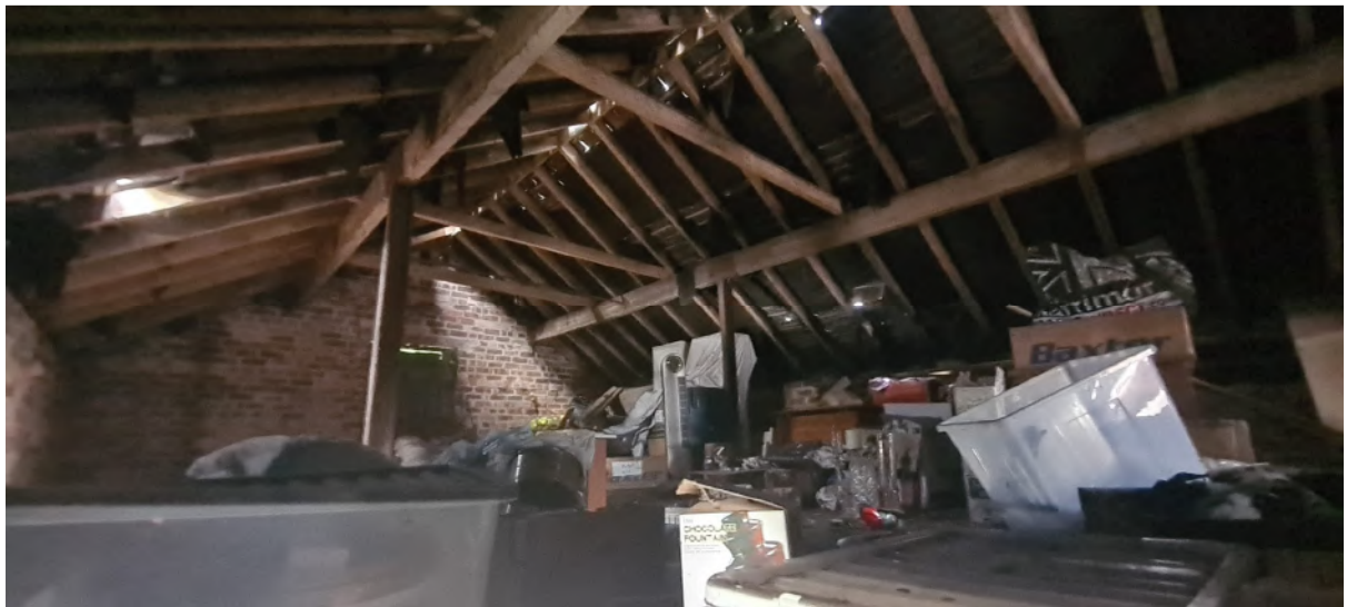
Fig 8. View internally of the 1 st floor showing timber posts and raised ties supporting the roof.
