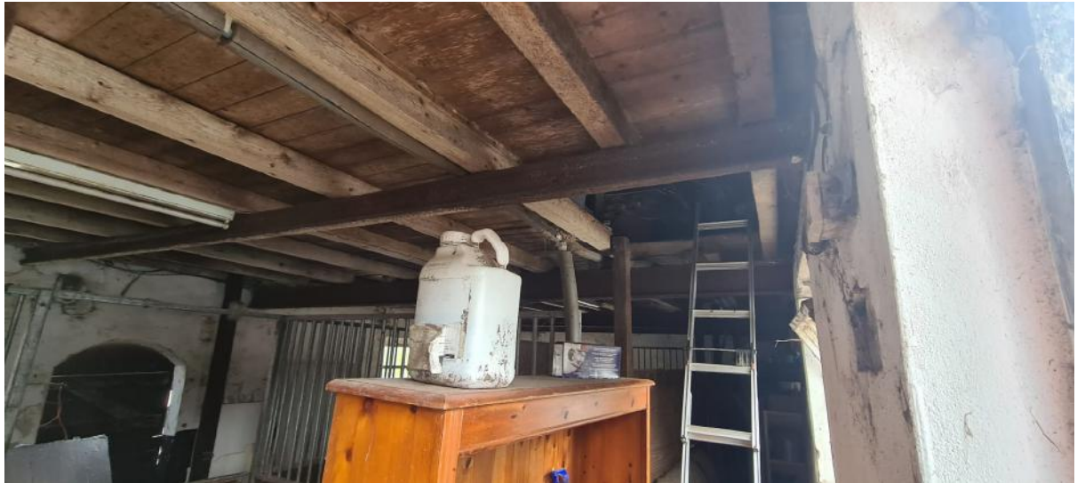
Fig 7. View internally of the ground floor showing steel beams and floor joist arrangement.
