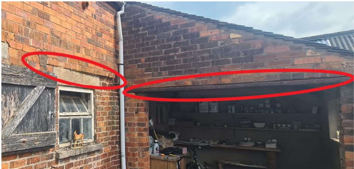
Fig 2. Corbelled brickwork over concrete lintel and steel railway track section over store room entrance.
