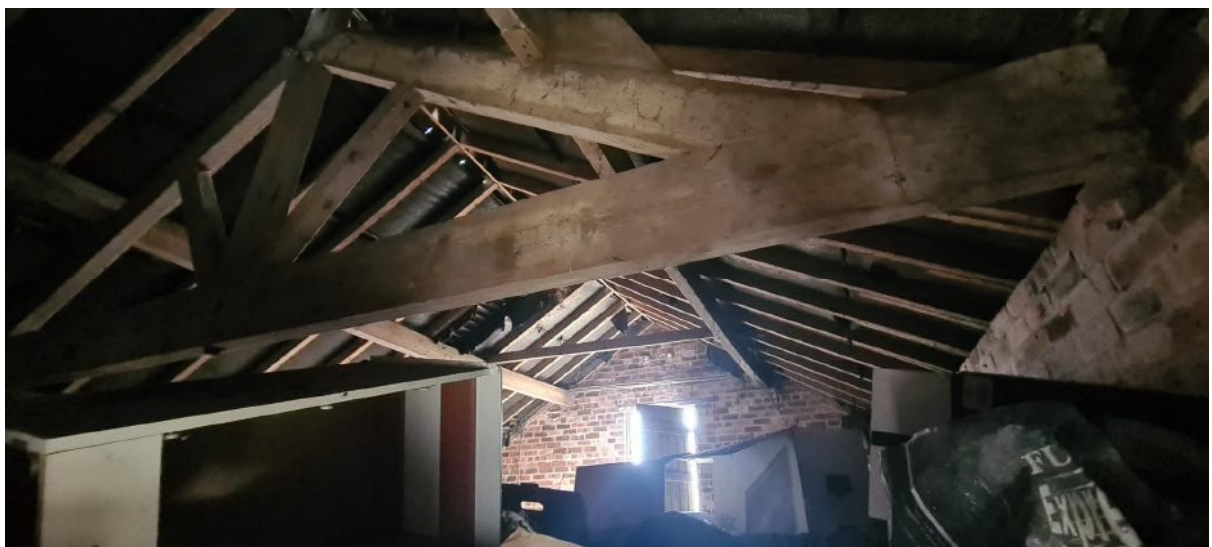
Fig 9. View internally of the 1 st floor showing kingpost truss supporting purlins within the roof.
