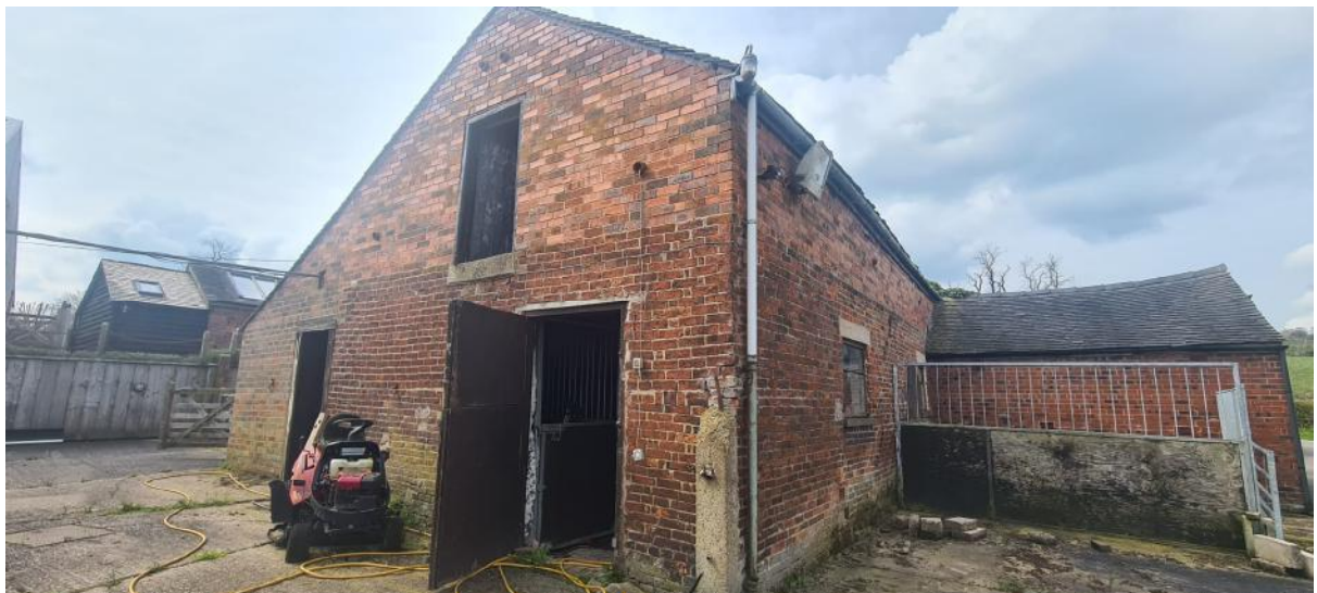
Fig 4. View of rear and left hand elevation.
