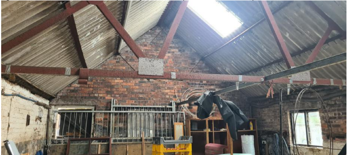
Fig 14. Internal view of steel fink roof truss and steel purlins.
