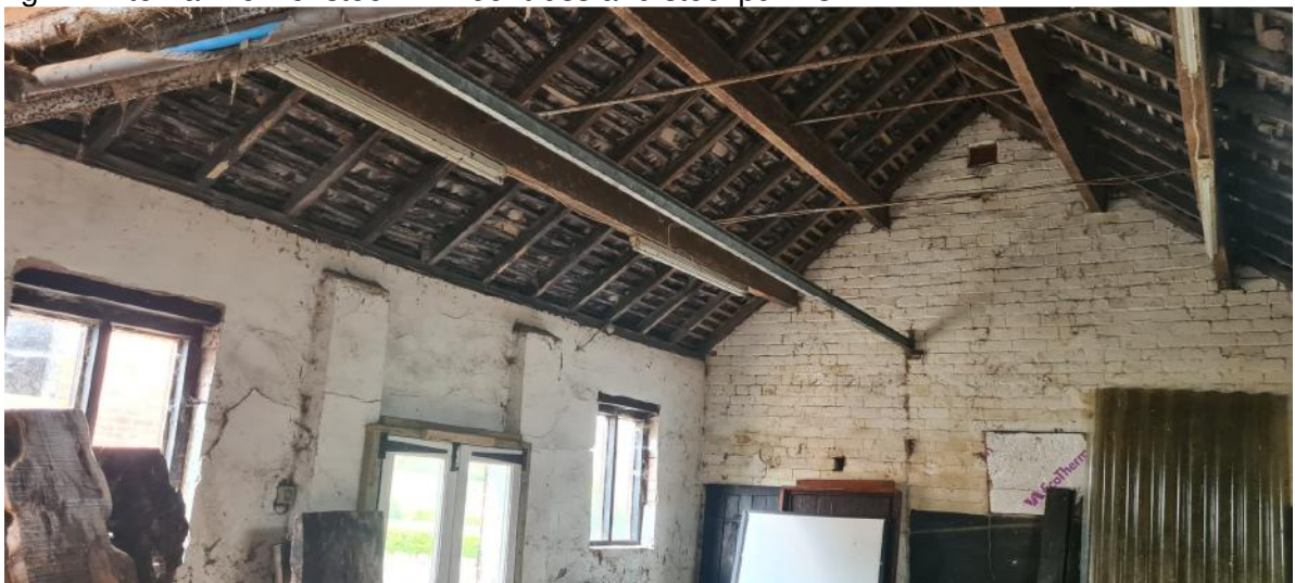
Fig 15. Internal view of timber purlins with steel rod ties.
