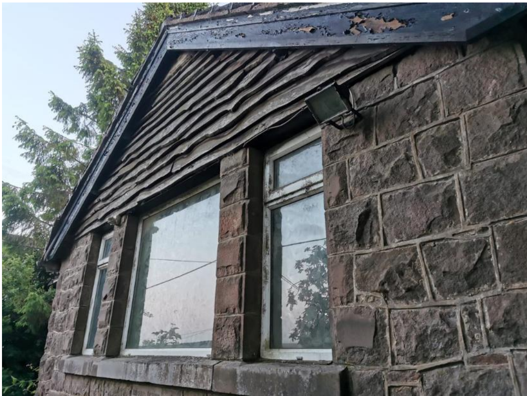
Plate 2: Photograph of the rendering present on B1 .
