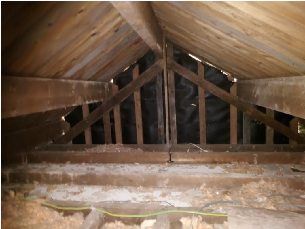
Plate 6: Further image of the internal void of B1 , showing how one half of the roof is lined with bitumen felt (right), and the other with timber sarking (left).
