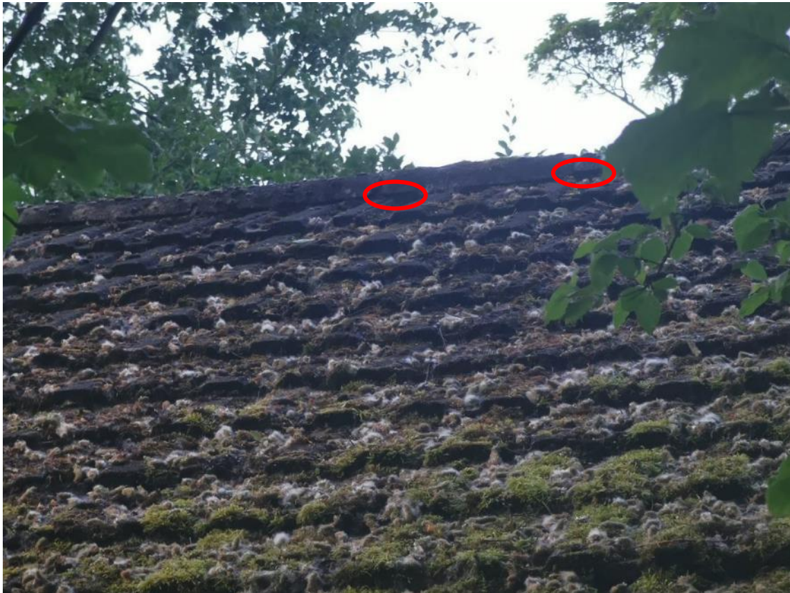
Plate 4: Evidence of the gaps at the ridge of B1 (circled in red).
