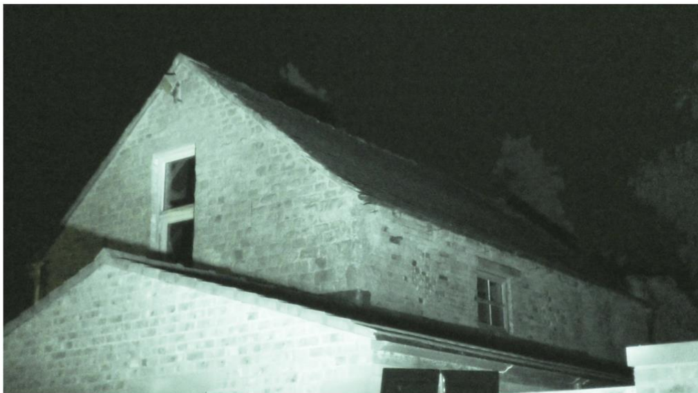
Image 2: NVA screen shot of northwest facing side aspect of building
