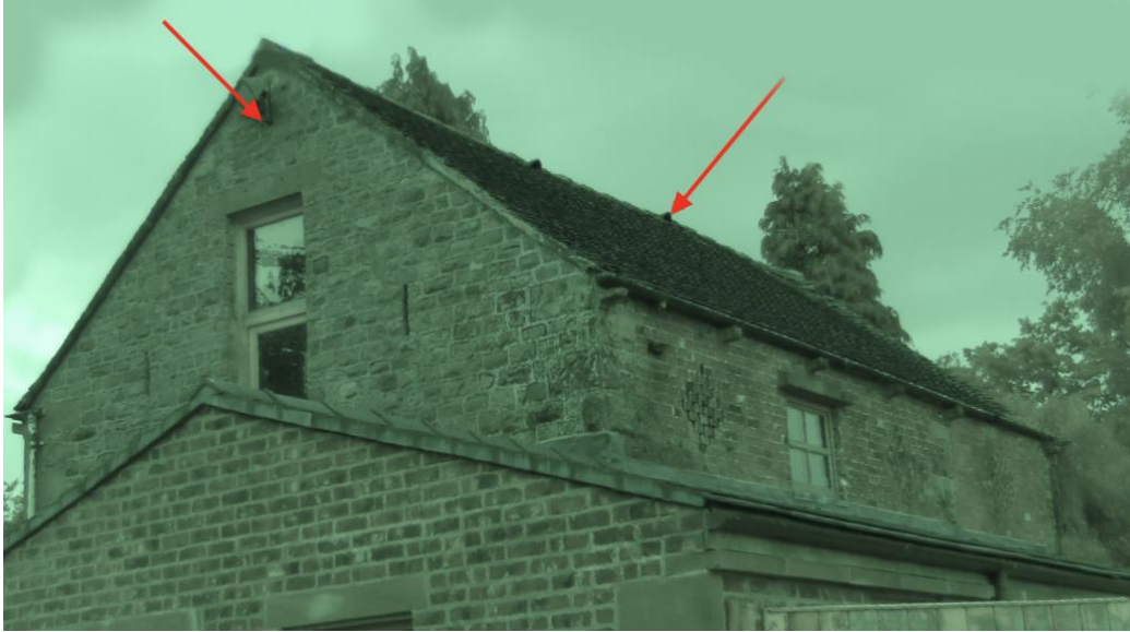
Image 3: red arrows point to roost access points via northeast facing gable wall and end ridge tile access
