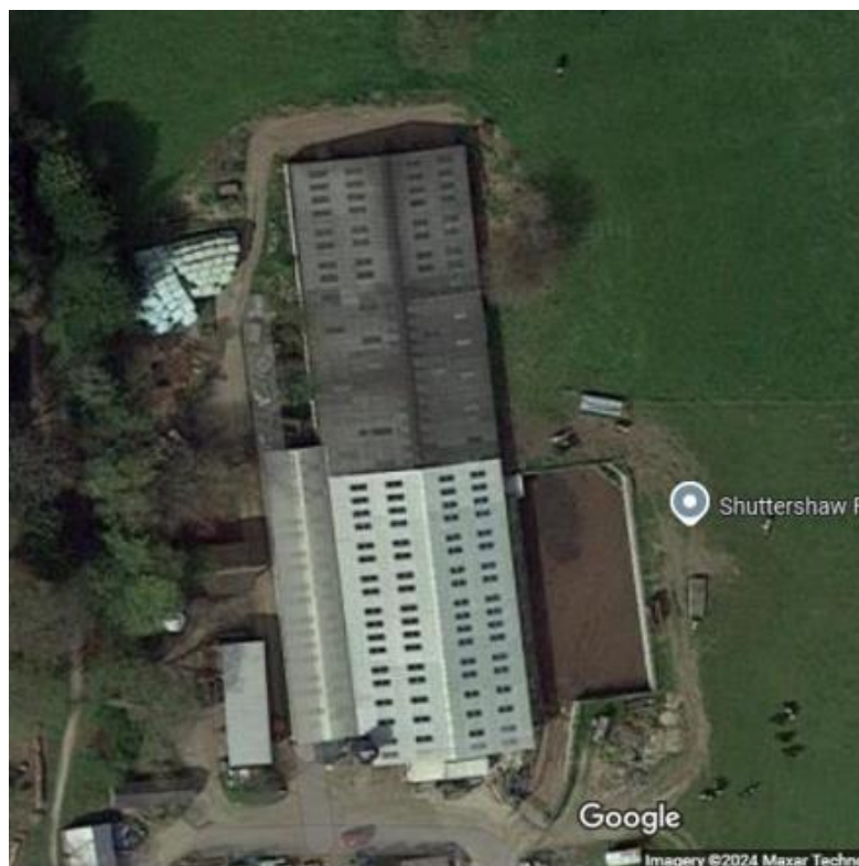
Figure 1 – Aerial image of proposed development site
