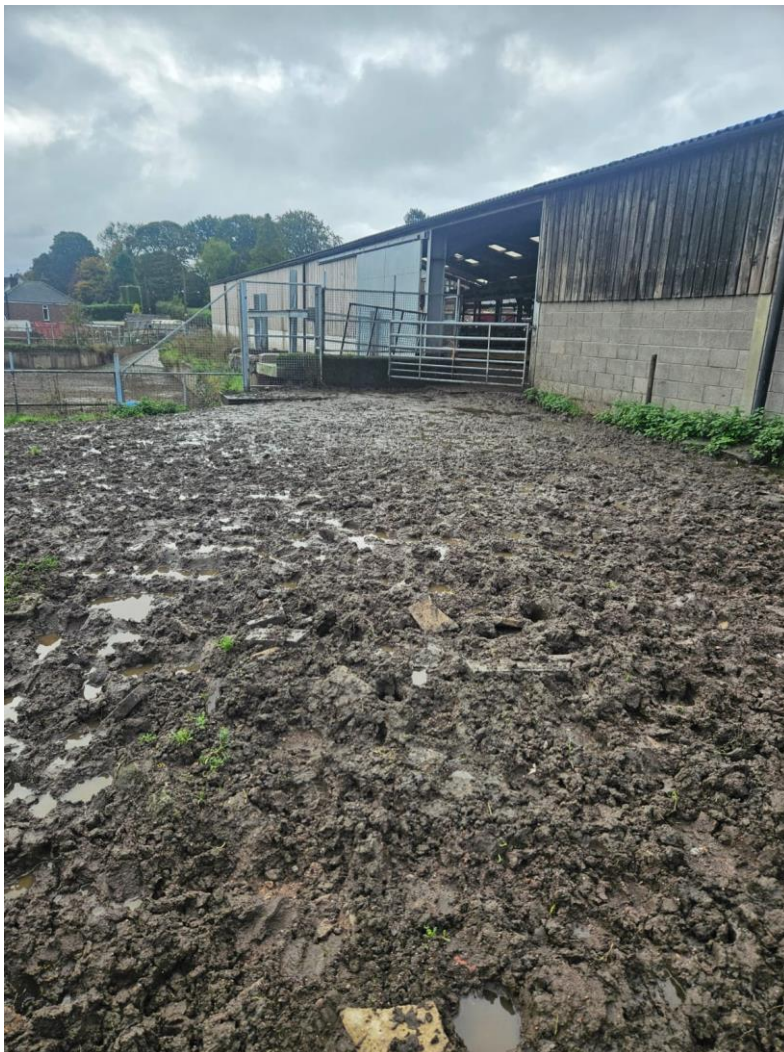
Photograph 1 – Proposed location of slurry tower
