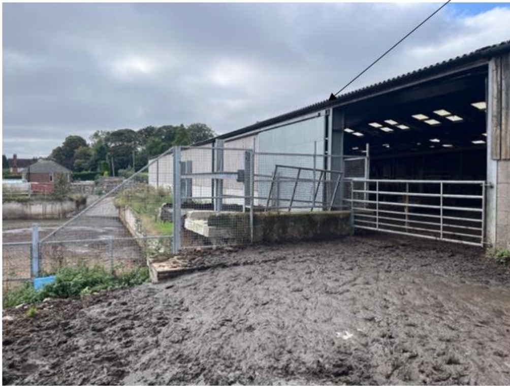
Photograph 2 – Proposed location of slurry tower adjacent existing cubicle shed
