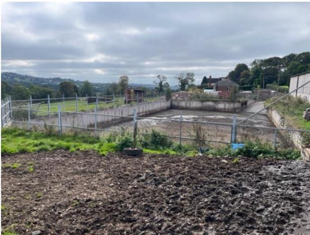
Photograph 3 – location of temporary access route to slurry tower to the north of lagoon.
