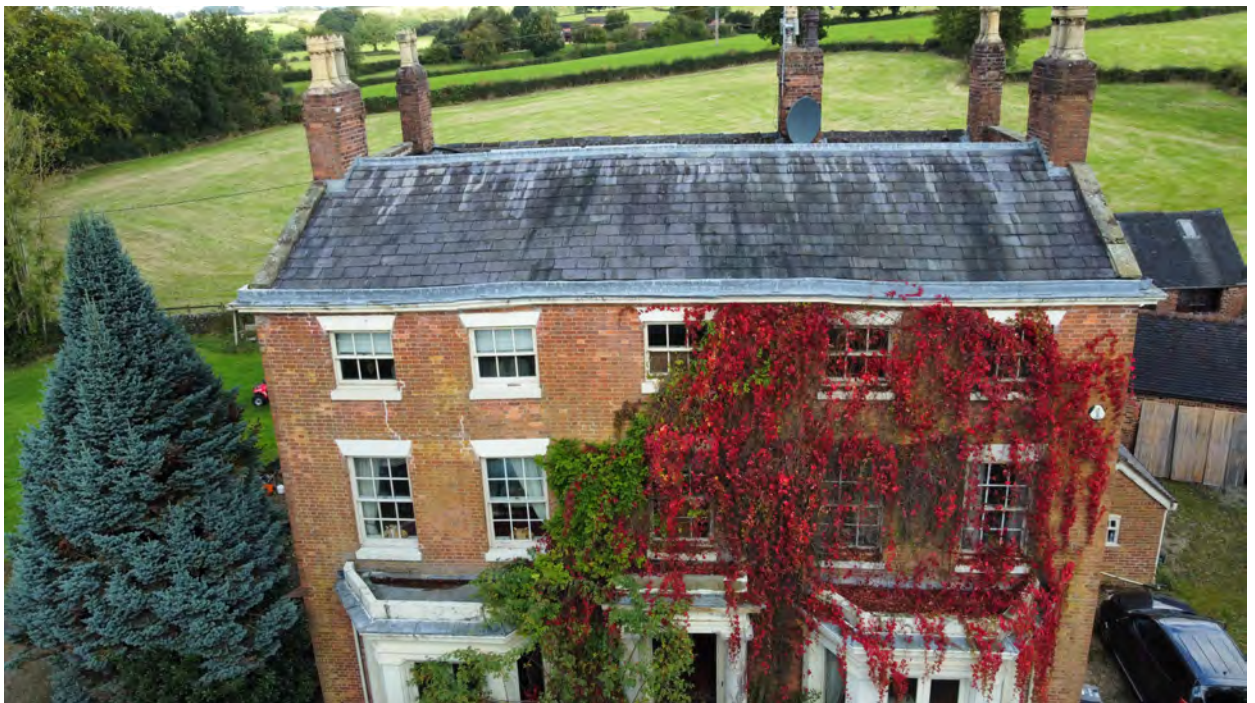
Plate 5. Drone image of the front pitch of the southern roof range.
