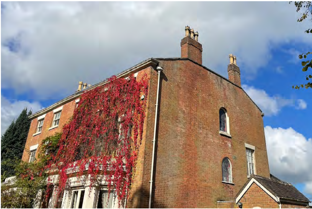
Plate 3. The eastern elevation of the AB showing the raised parapet wall.
