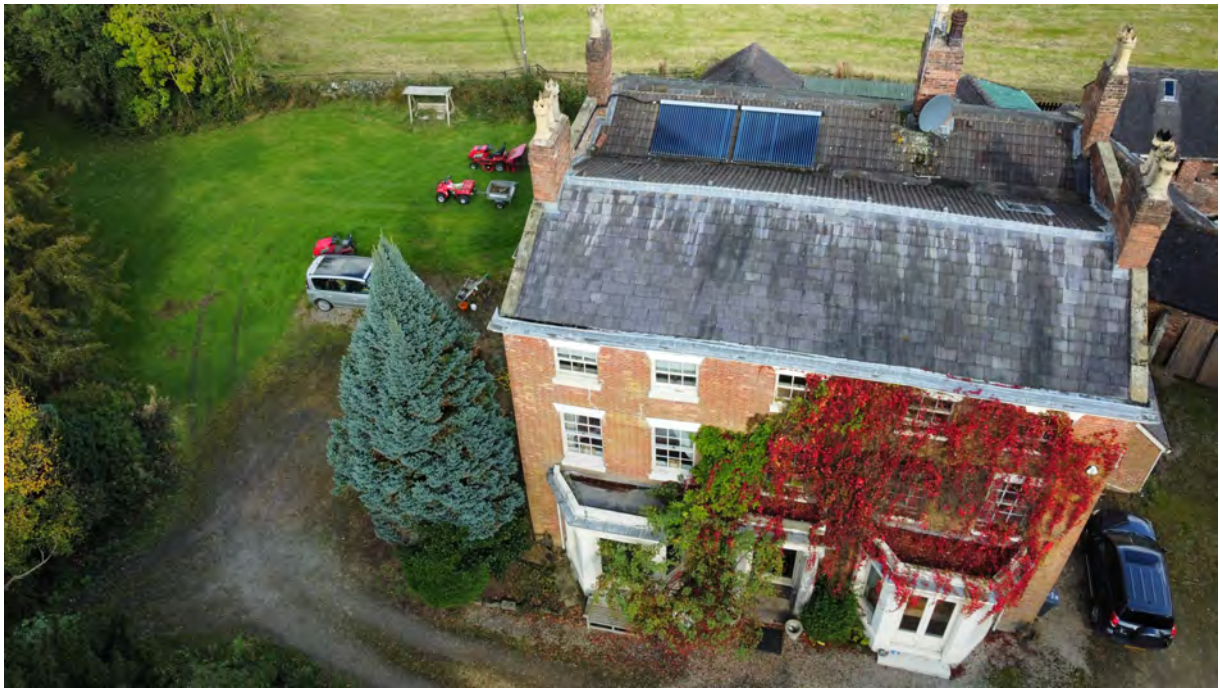
Plate 6. A bird's eye view of the roof of the AB.
