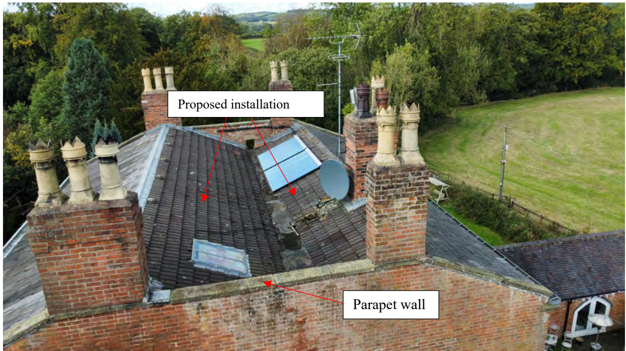
Plate 4. View of the two parallel roofs on the AB.
