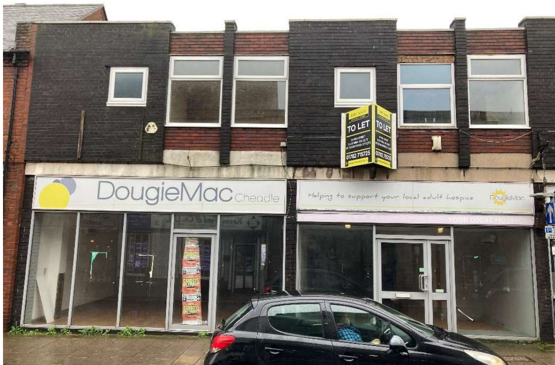
Figure 1: Photo of the 26 High Street, Cheadle, as existing, features one public facing façade.
