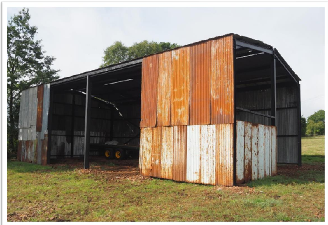
Figure 2: Application building - DET/2022/0043
