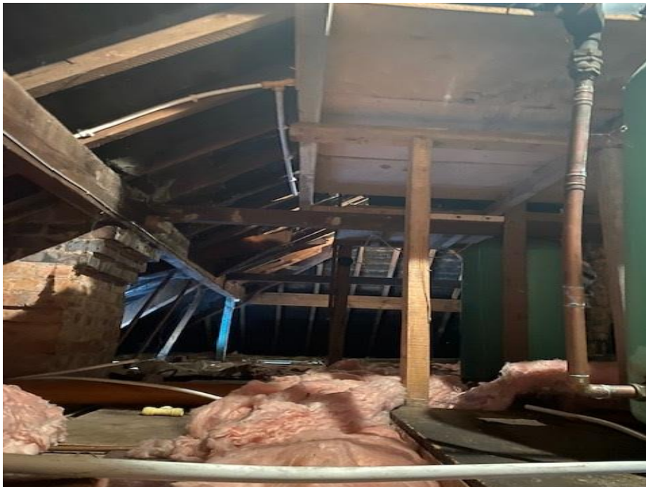
Figure 8. View of loft space (Grid ref: SK 04956 42054)
