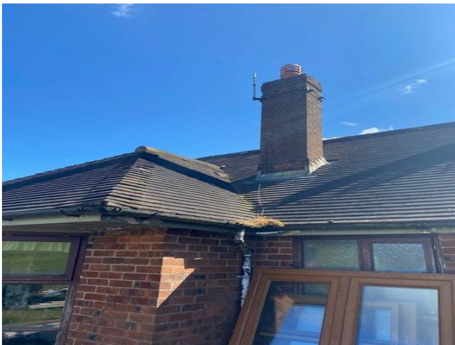
Figure 92. View of northern chimney and hipped roof (Grid ref: SK 04948 42058)
