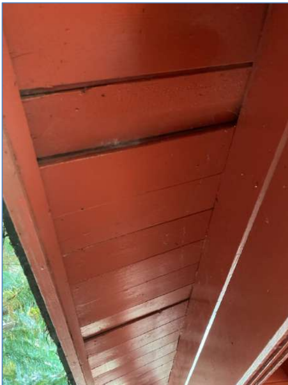
Figure 6. Potential access into soffit box/ internal cavity
