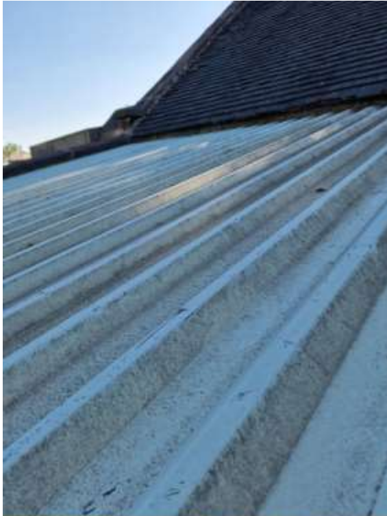
Corrugated roofing on east side single storey building
