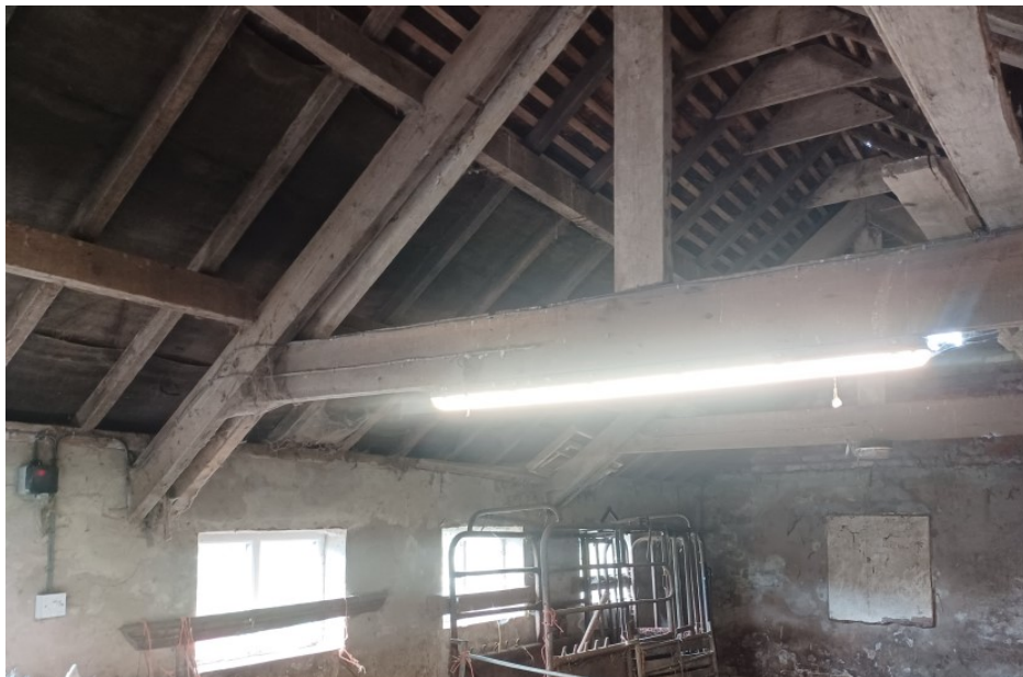
Photo 6: View of truss
