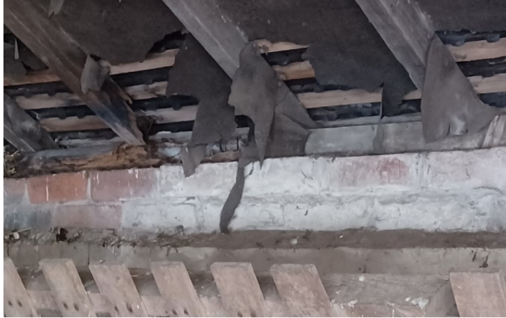
Photo 7: Damaged wallplate
