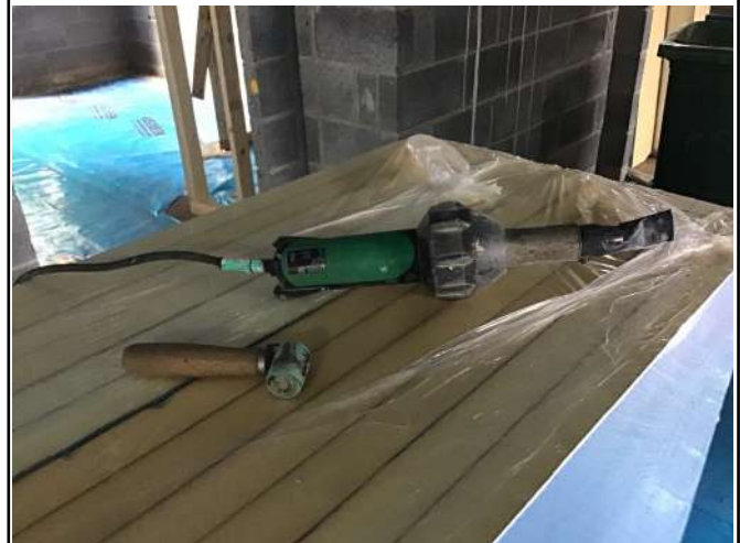
Heat source being used.
