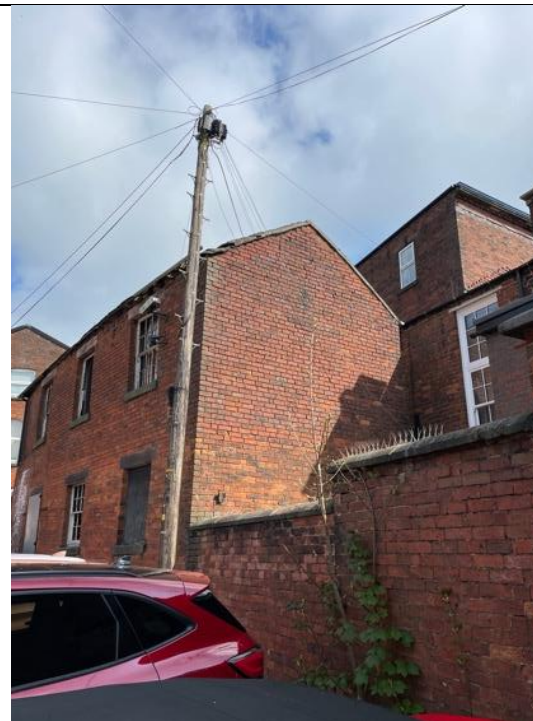
Photograph 4: South facing aspect of Area A
