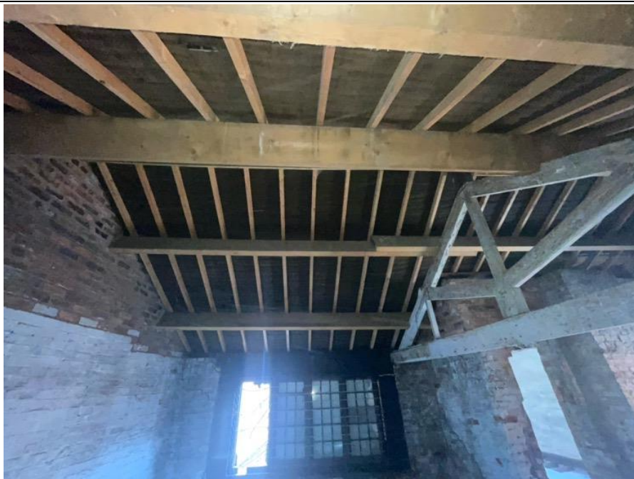
Photograph 9: Recently replaced roof of Area B
