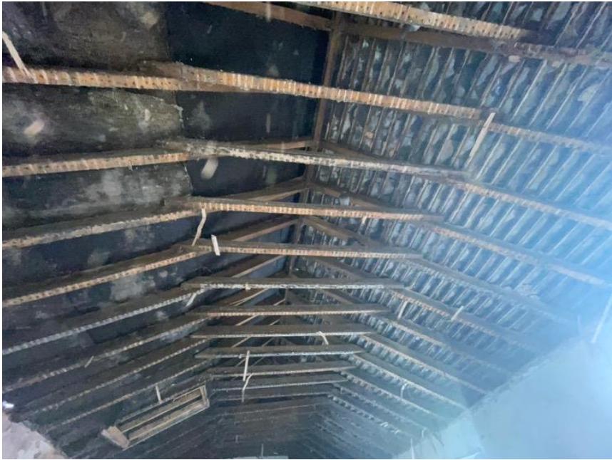
Photograph 8: Removed ceiling showing tile covering (Area A)
