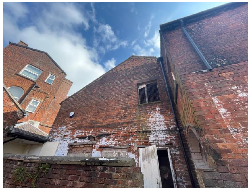
Photograph 6: West facing aspect of Area B
