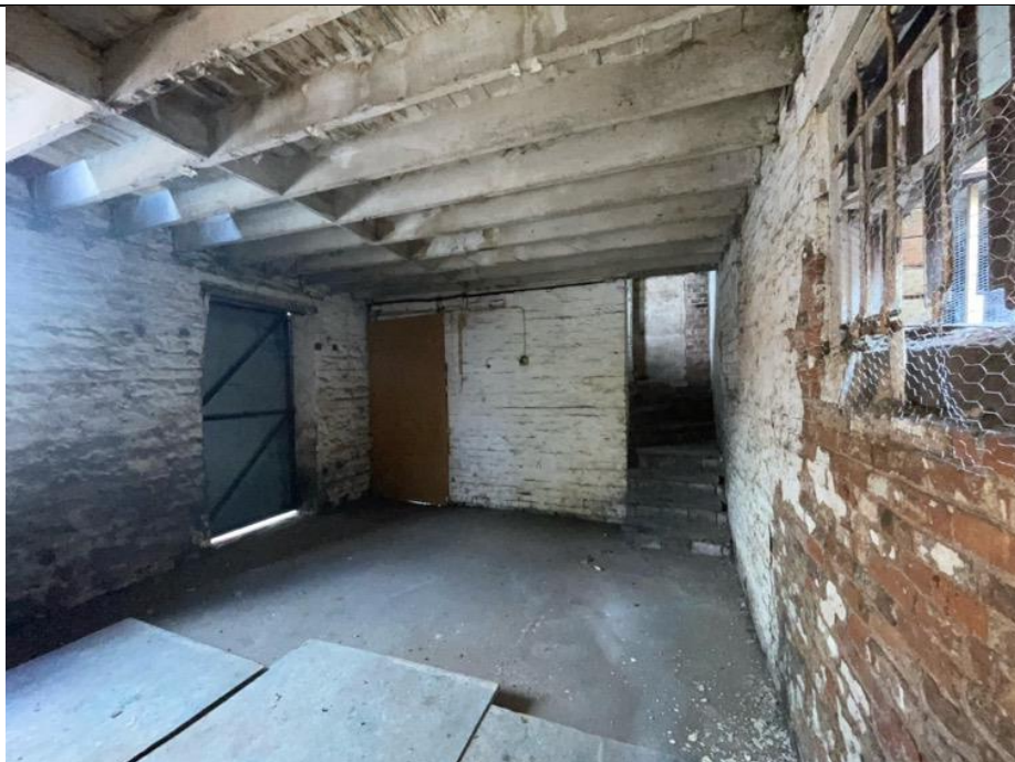
Photograph 5: Ground floor of Area A
